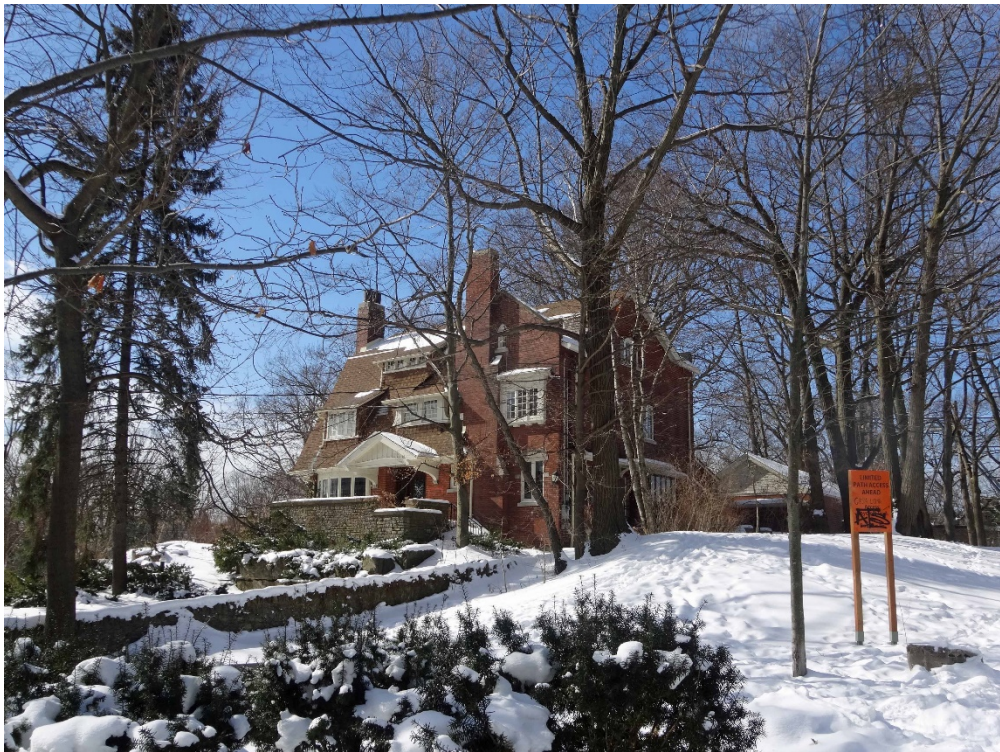
Views of the principal (east) elevation (above) and the context from Russell Hill Road (below). Photograph: Heritage Preservation Services, 2019
