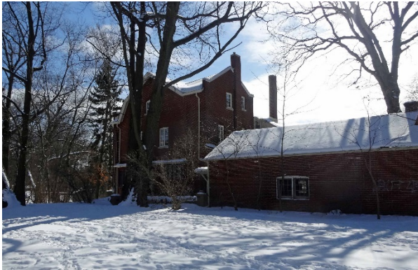
4c. rear (west) elevation (right);
