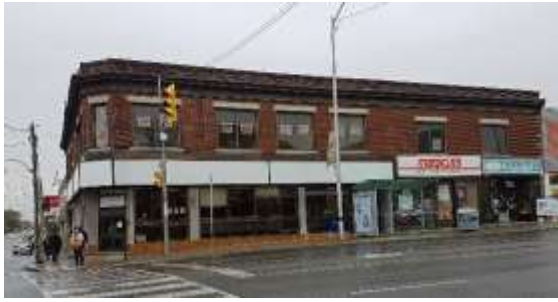
4a. South elevations of 2078 (left) and 2086 Danforth Avenue
