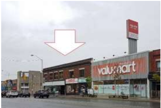
4c. Contextual view, looking west on Danforth Avenue to Woodbine Avenue and showing the subject properties anchoring the northeast corner of the intersection
