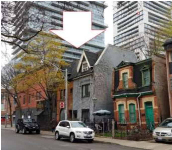
Contextual view east on Granby Street, showing the subject properties between the listed heritage properties at 77 Granby (right) and 414-418 Church Street (left)
