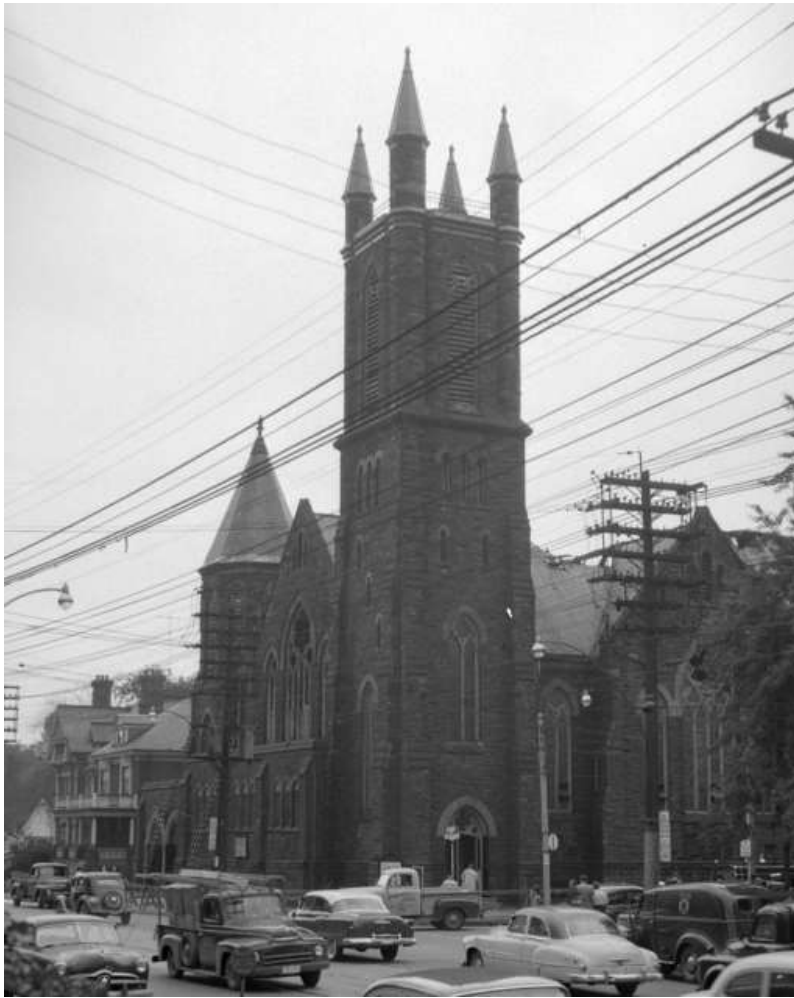
31. "Aftermath of the Fire" at Bloor Street United Church, August 1954 – the photograph shows the damage to the roof and the stained glass windows. The photo also shows the removal of the steps on Bloor Street and the replacement of the three arched openings with the row of 9 arched windows following the widening of Bloor Street in 1927. The arches can be seen in the single storey pavilion which was relocated to the west. (TPL, James Victor Salmon collection, S1-2029B)
