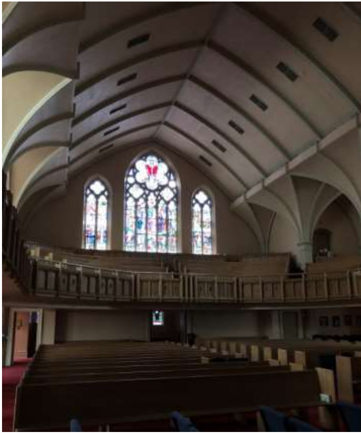
42. Interior looking south showing the new structure of the columns, arches and ceiling (HPS, 2019)
