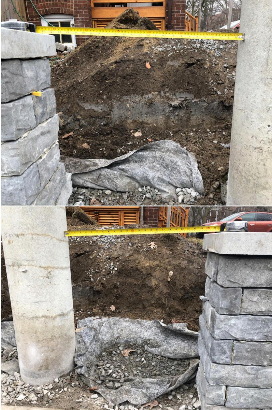
Records Services, Engineering Services
