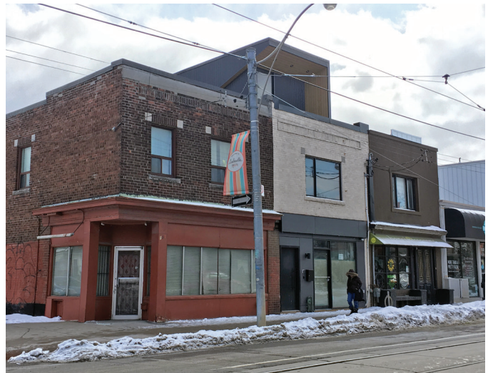
Example of a well-integrated one storey addition to a low-rise building.
