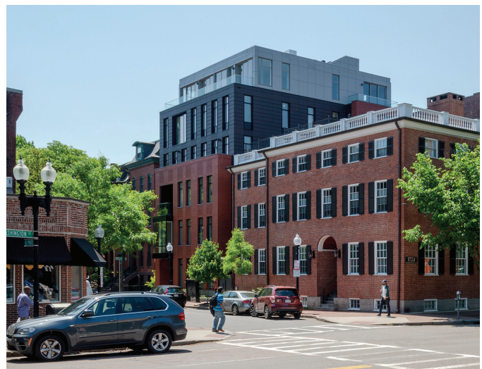
The base of a six-storey building is designed to reference the horizontal datum line of the adjacent three storey building by using similar materials and aligning the height of the building base. Upper storeys are stepped-back and differentiated in the material and colour choice while respecting the architectural rhythm with the placement of the window openings. Credit: Utile, Inc., Boston Photo by: Ryan Maheu Photography
