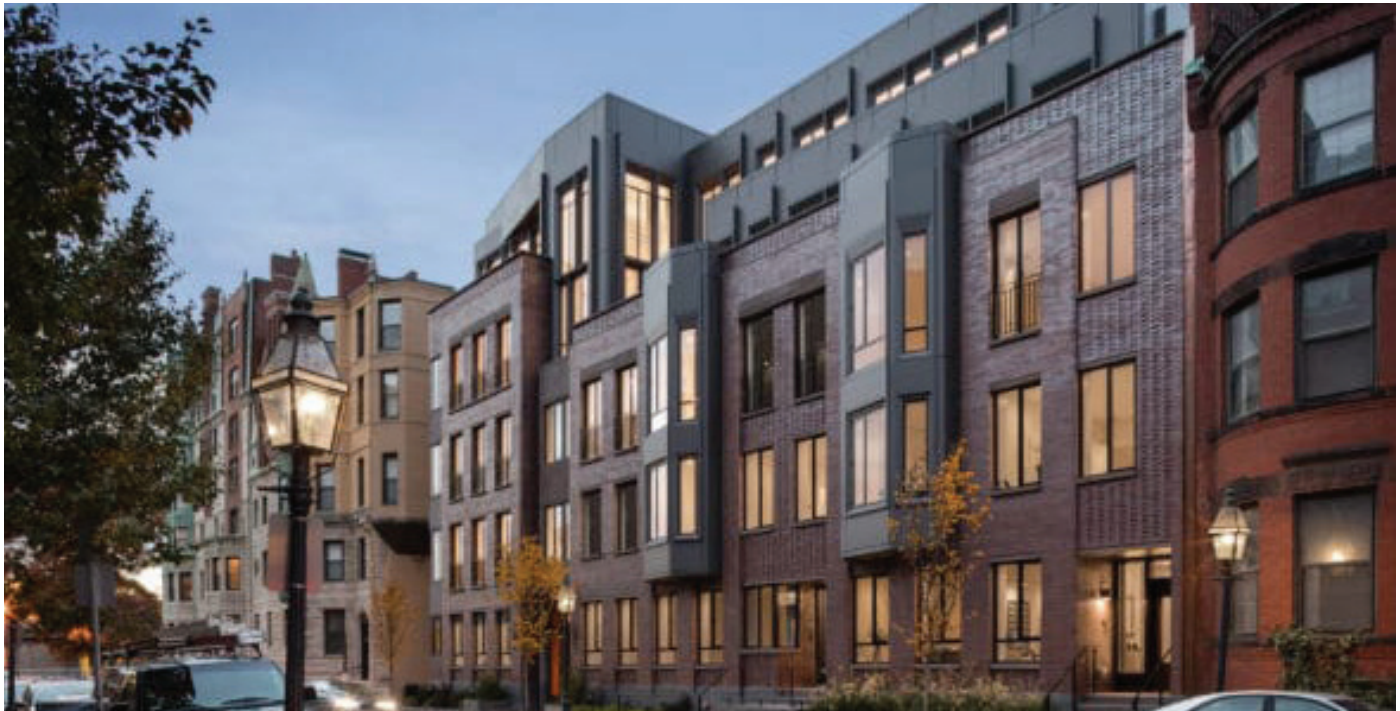
A good example of a building with a well-designed facade along the street frontage with vertical rhythm, bay windows, and articulation. Carefully designed brickwork, subtle variations in facade depth all help to reduce the visual bulk of the building. Credit: Hacin + Associates, Boston Photo by: Trent Bell Photography
