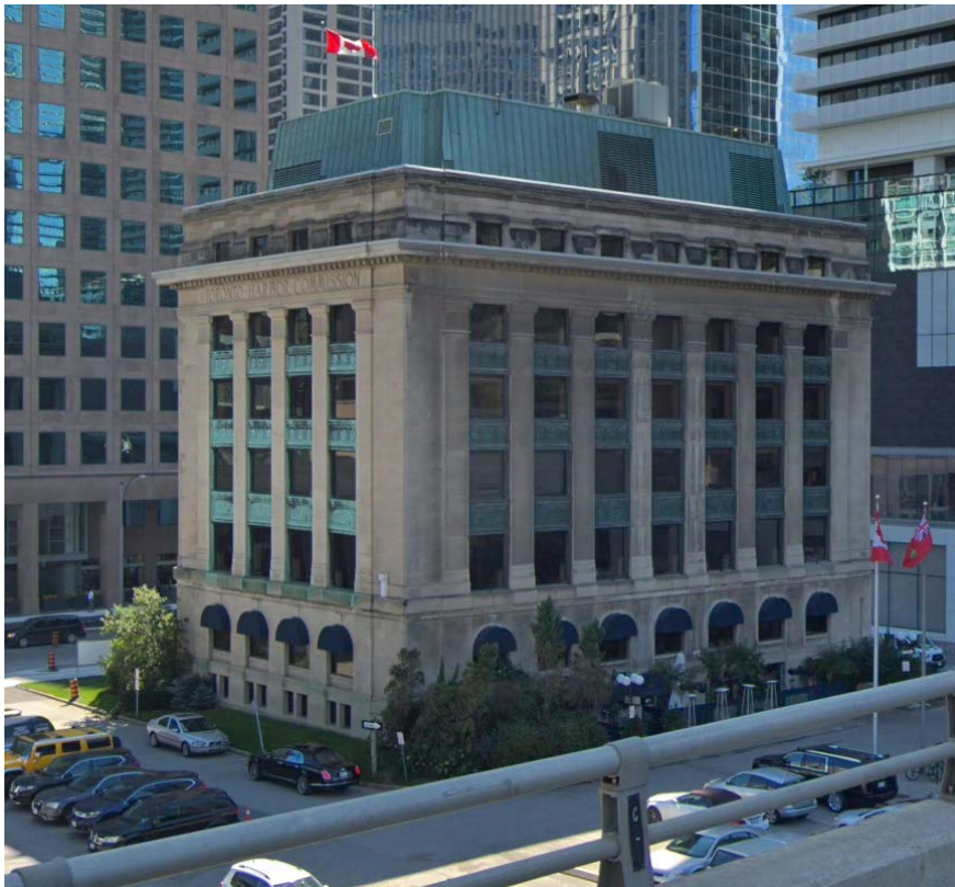
East (left) and north (right) elevations of 30 Bay Street
