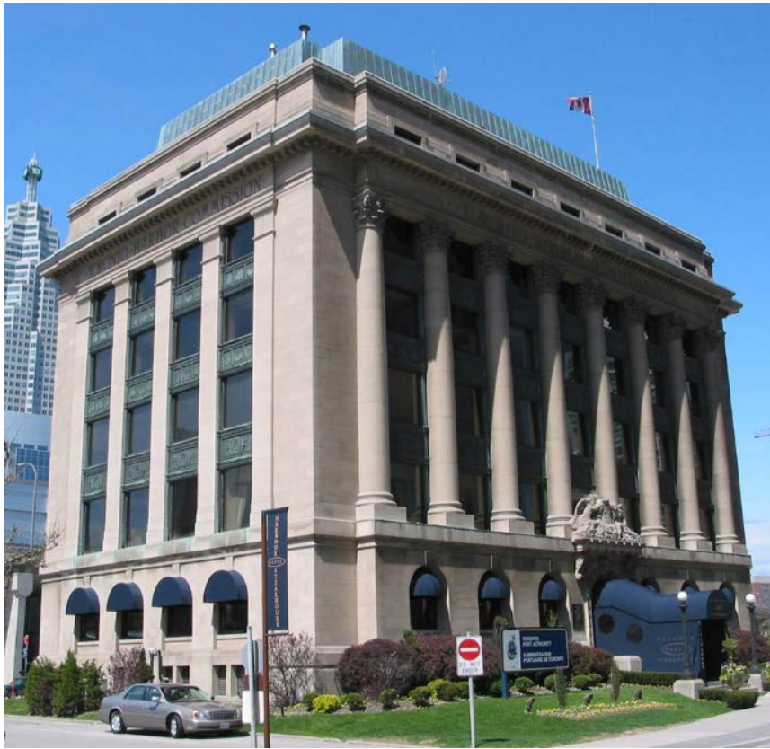
West (left) and south (right) elevations of 30 Bay Street
