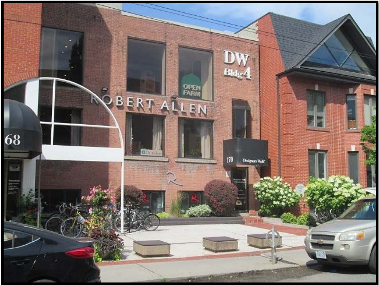
Attachment 'B' – Photo of proposed parking site – 170 Bedford Road
