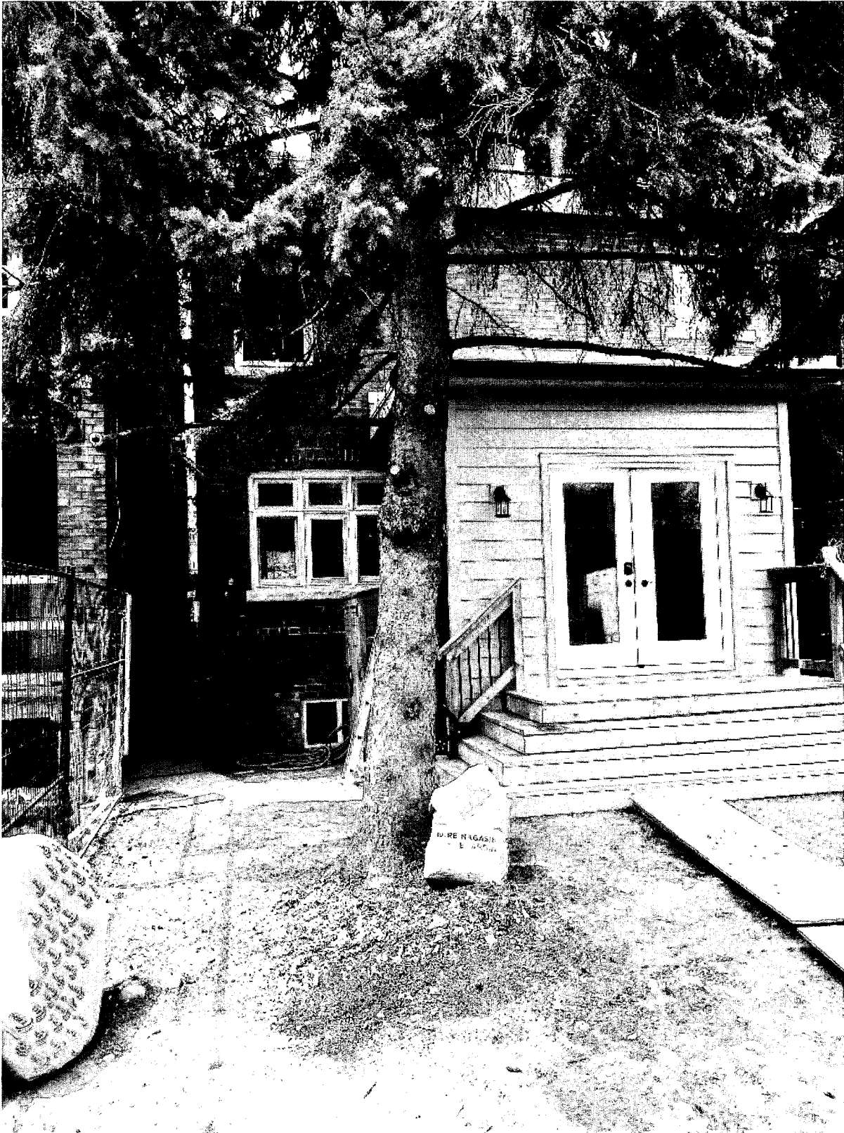
Figure 2: May 15, 2019 TPRR staff photograph of the white spruce in relation to the dwelling, the newly installed rear deck at 175 Walmer Road, and ongoing construction occurring at 173 Walmer Road.
