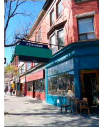
Low-rise, main street character retail buildings that are historically connected with Harbord Village to the north
