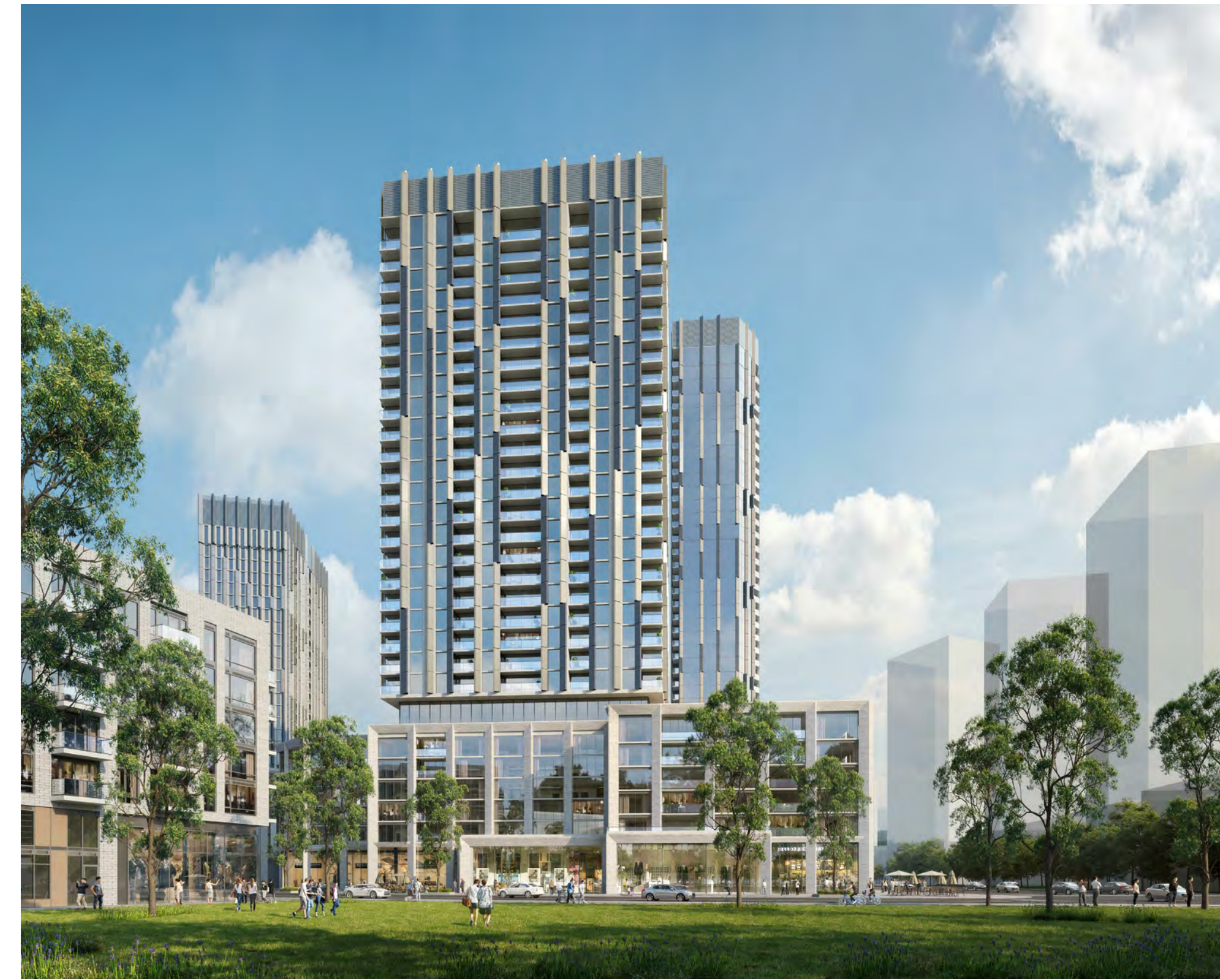
1 NORTHWEST CORNER VIEW AT DEDICATED PARK A461.S
