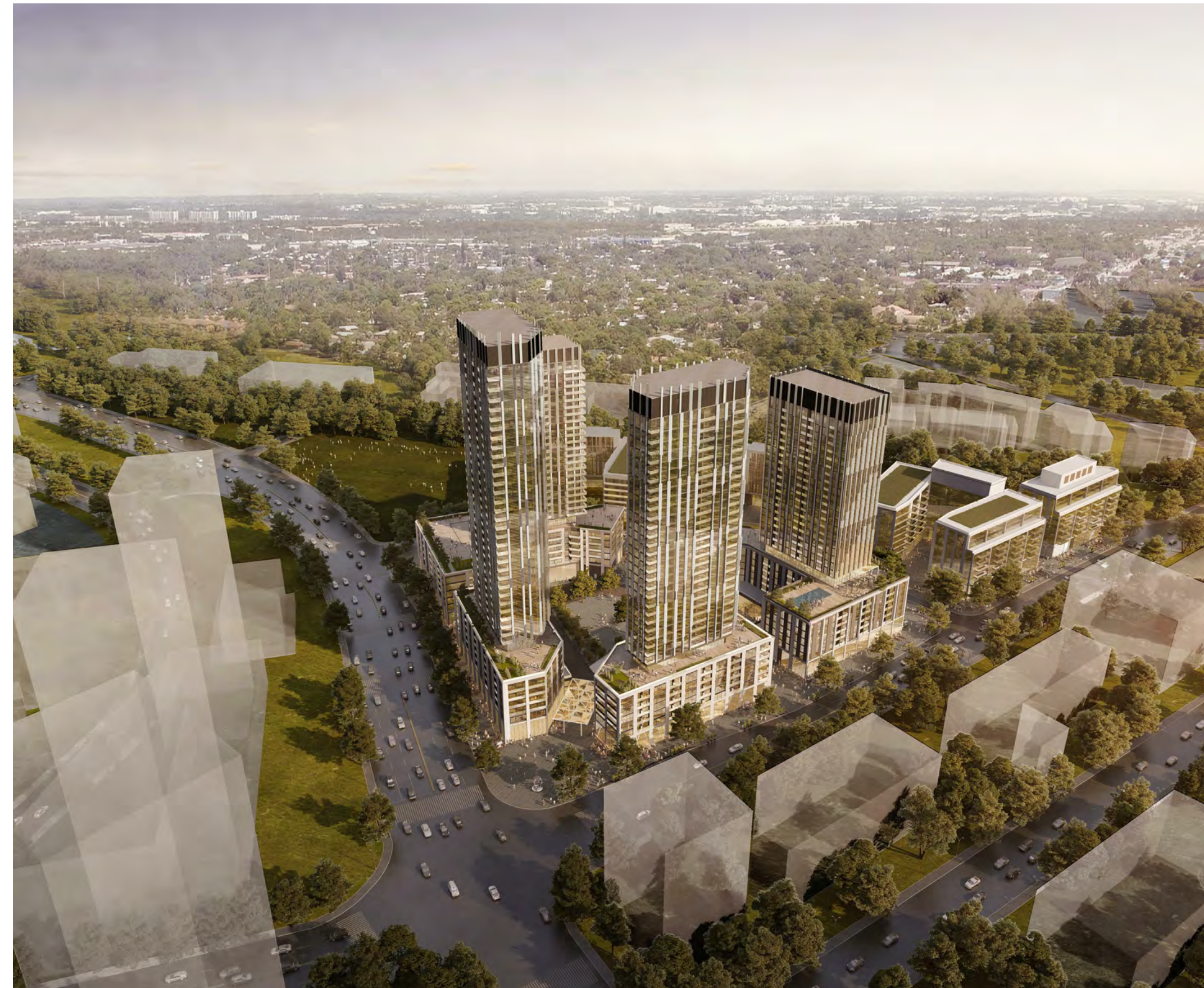
4 AERIAL SOUTHEAST CORNER VIEW A461.S
