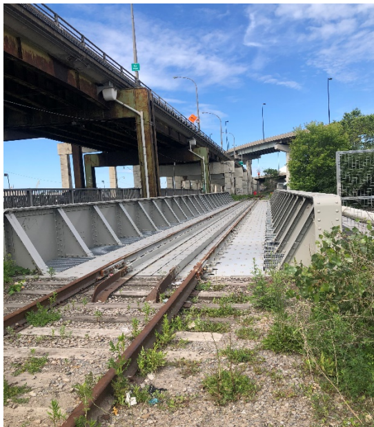
Picture of the Bridge, looking west
