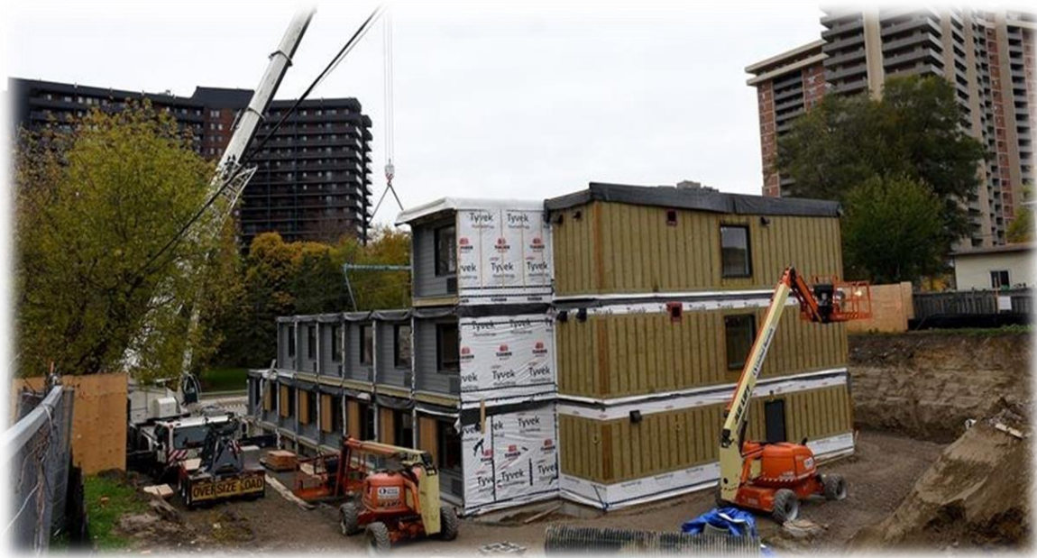
Construction progress as of October 28, 2020
