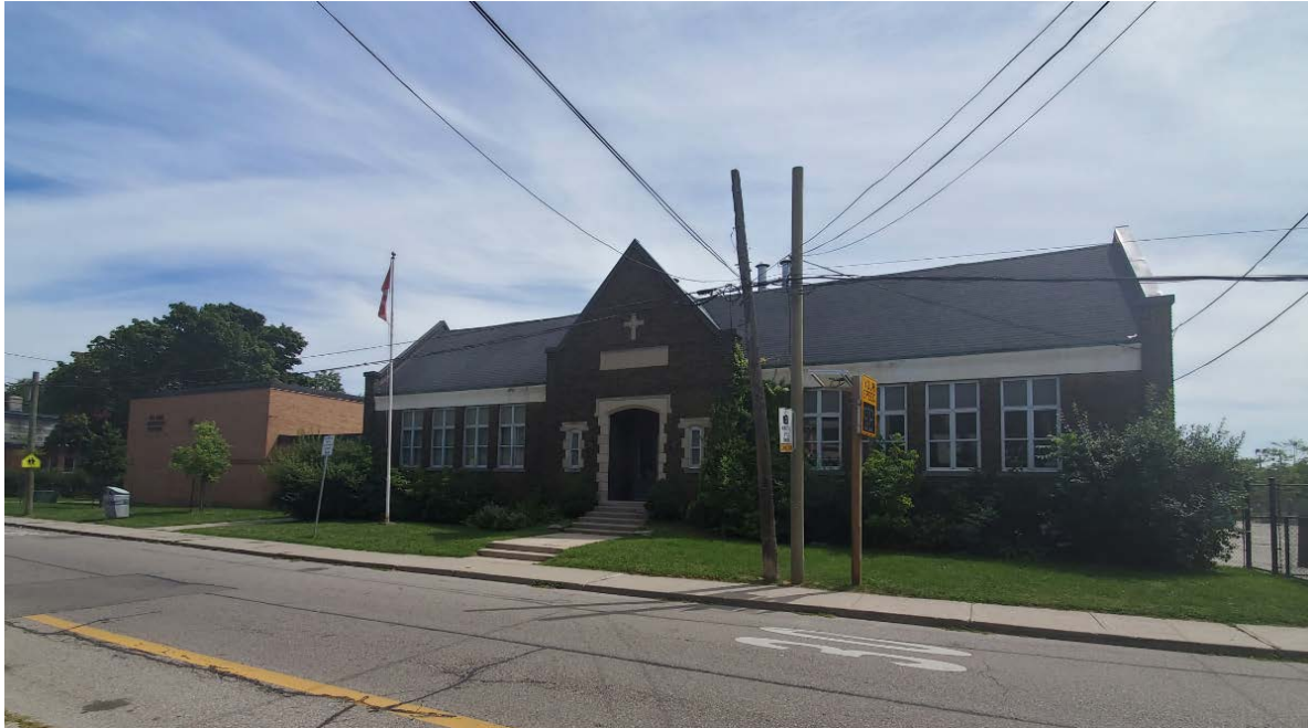
Detail of the principal (north) elevation of St Leo's Catholic School, showing the original 1926 building (right) and the 1976 addition (left) (Heritage Planning Image, 2020)
