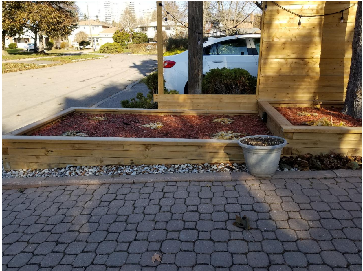
Attachment 5: View of section of fence removed by property owners at 52 Axsmith.
