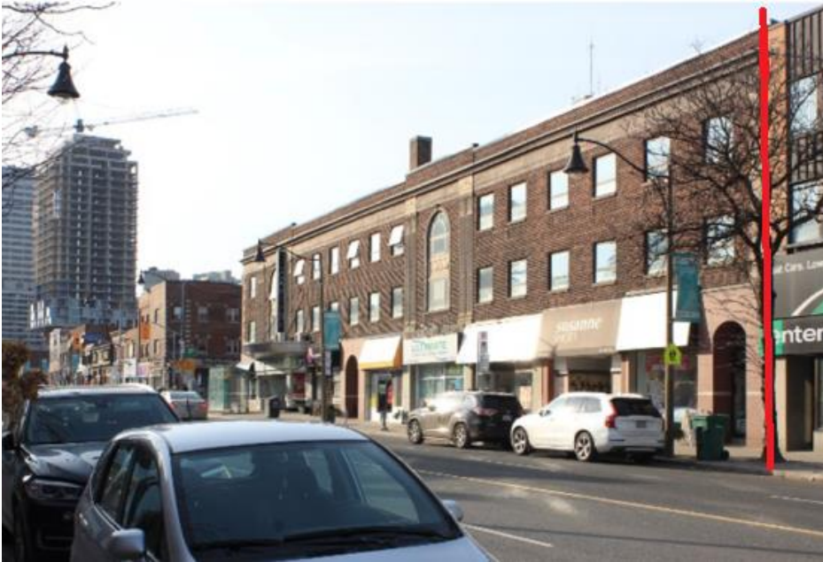
View (facing southwest) of the existing property's primary east elevation with a red line indicating the northern boundary of the heritage building
