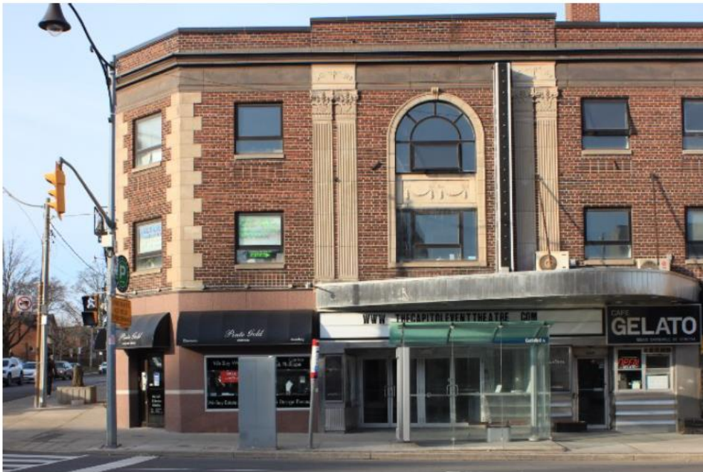
View (facing west) of the primary east elevation of the existing property, including the Art Deco-style theatre marquee and entrance
