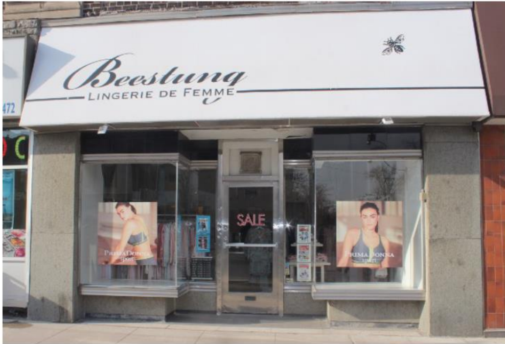
View (facing west) of the primary east elevation of the existing property, including the Art Deco-style storefront at 2504 Yonge Street
