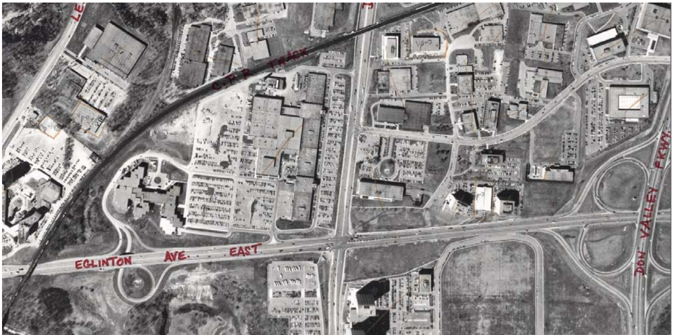
Plate 117, Series 12 Aerial Photographs of the Metropolitan Toronto Area, 1971: showing the completion of the pre-planned extensions at the west and north-west corners of the Former IBM (Canada) Headquarters building at 1150 Eglinton Avenue and the large extension to the rear of 844 Don Mills Road as shown in the plan drawing below. Note that the lawns on Don Mills Road have been replaced with parking. (CTA)
