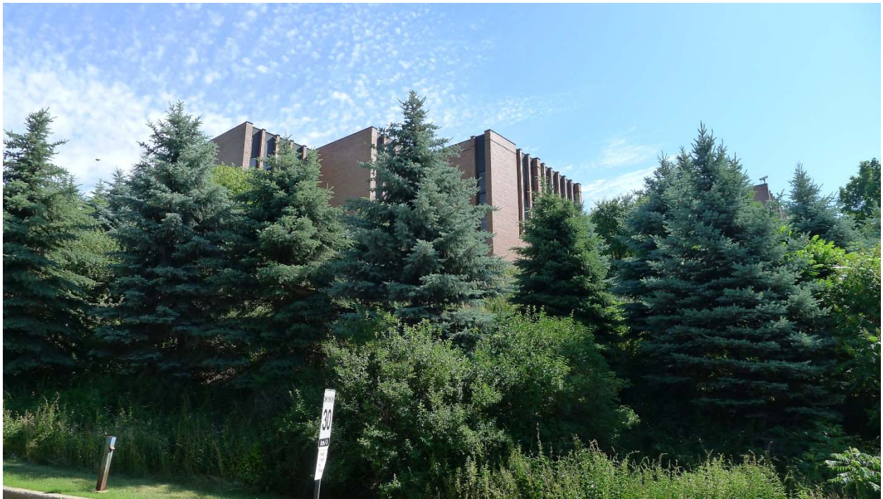
The Former IBM (Canada) Headquarters building: viewed from the driveway from Eglinton Avenue East (HPS, 2016)
