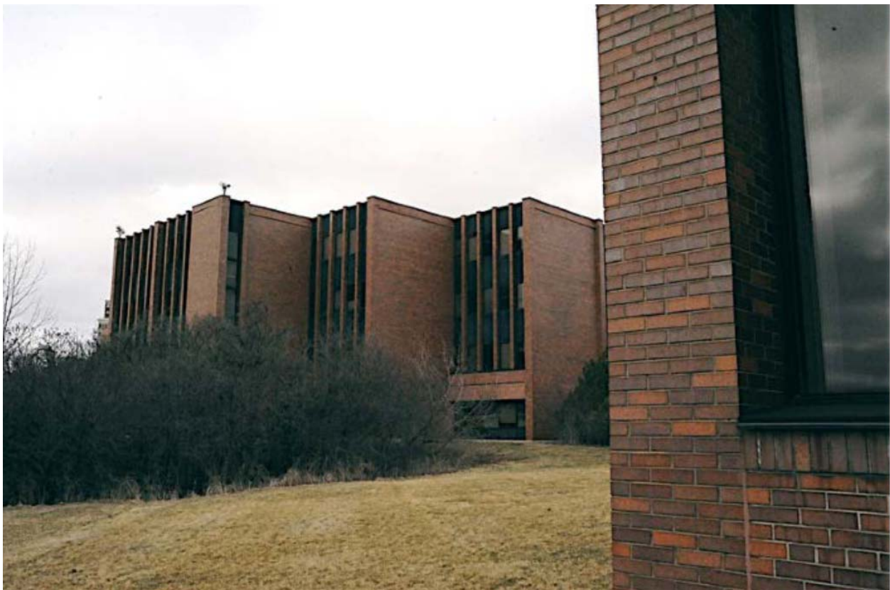
1150 Eglinton Avenue East (Source: Goldsmith Borgal & Company Ltd. Architects, February 13, 2018) - Partial view of the south elevation
