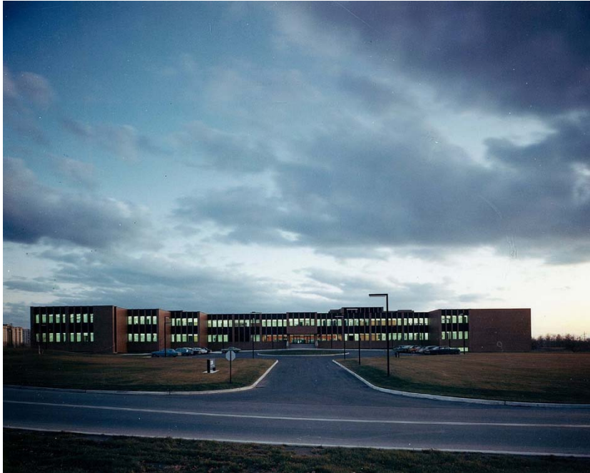
The Former IBM (Canada) Headquarters building, North Entry Court 1966-67: showing the building prior to Phase 2 (Panda Associates, IBMhq-06, NORR Architects, Engineers and Planners)
