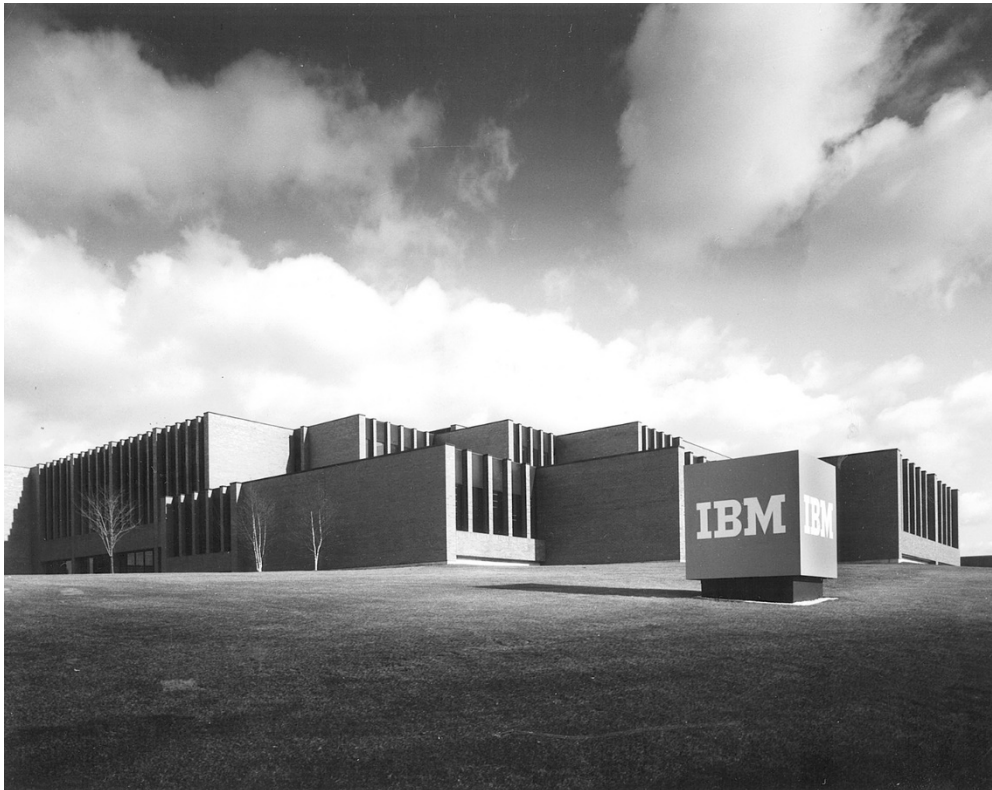
The Former IBM (Canada) Headquarters building: looking east with a view of the cube sign designed by Eliot Noyes (Panda Associates, IBMhq-04, NORR Architects, Engineers and Planners )
