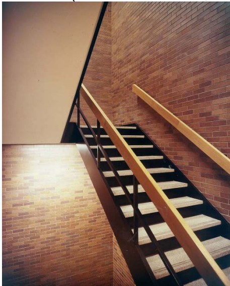
The Former IBM (Canada) Headquarters building: showing the staircase with the material palette of the exterior, brick and black metal continued inside. (Panda Associates, IBMhq-01, NORR Architects, Engineers and Planners)
