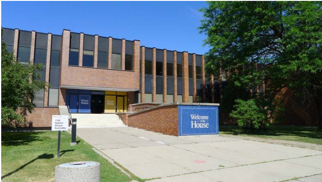
East Entry: showing the same arrangement as the north entry with the broad steps, recessed doors and cantilevered bay here modified with a ramp for universal access. The east elevation faces the parking lot but is set back in lawns with mature trees (HPS, 2016)
