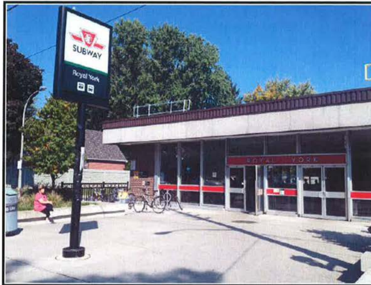
Royal York Subway Station
