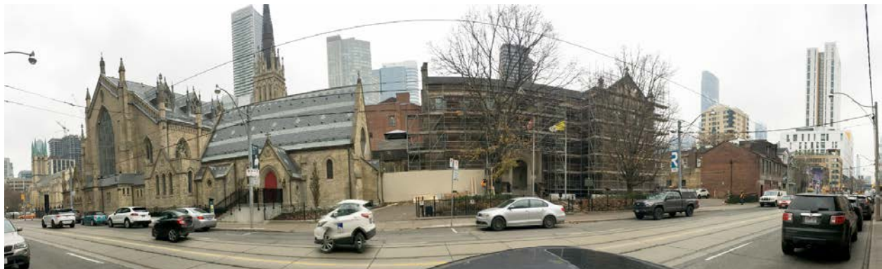
Adjacent West Side of Church Street (Opposite to development site)
