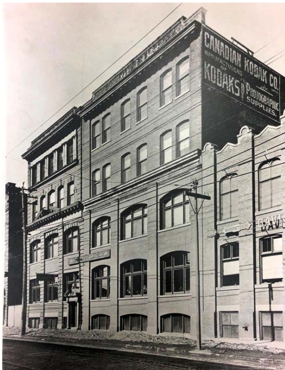
20. 582 King Street West, south elevation, 1912 (Ryerson University Library: Special Collections [RU])
