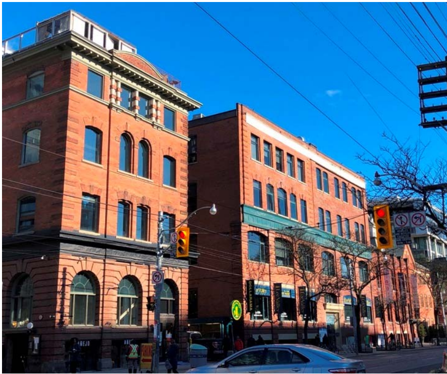
35. King Street at the northeast corner with Portland looking east at a strong collection of warehouse buildings including 600 King Street, 1900, 582 King Street West (aka 590 King Street West), 1902-1904, 580 King Street West (1904) and 570 King Street West (the Toronto Silver Plate Co. building, 1882) (HPS, 2020)
