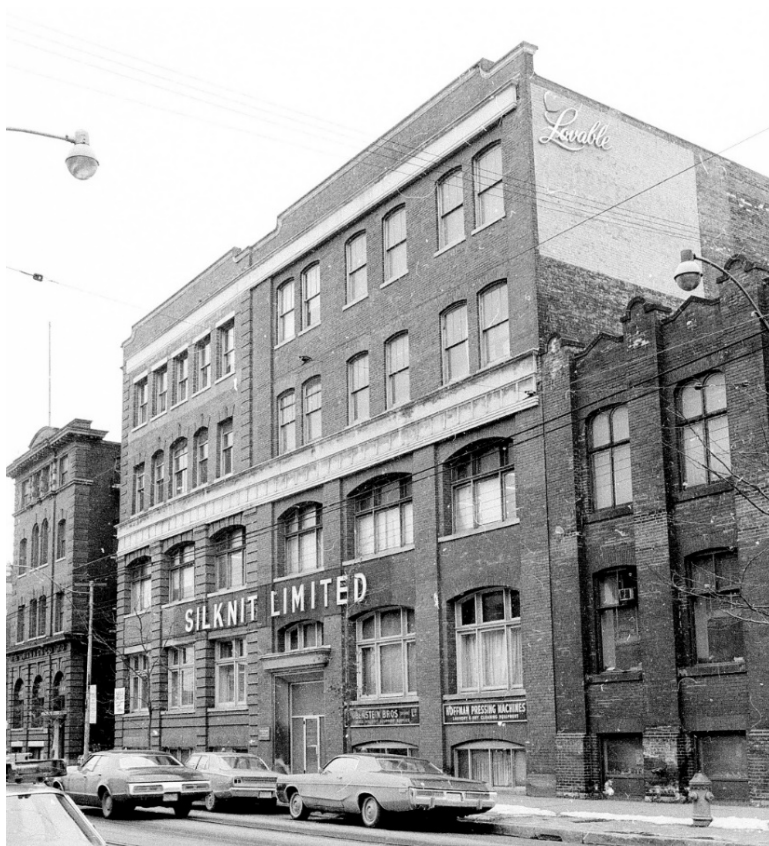
23. 582 King Street West, 1973 photograph showing the alterations undertaken by Silknit which relocated the door, removed the original door and many of the decorative stone elements. (CTA)
