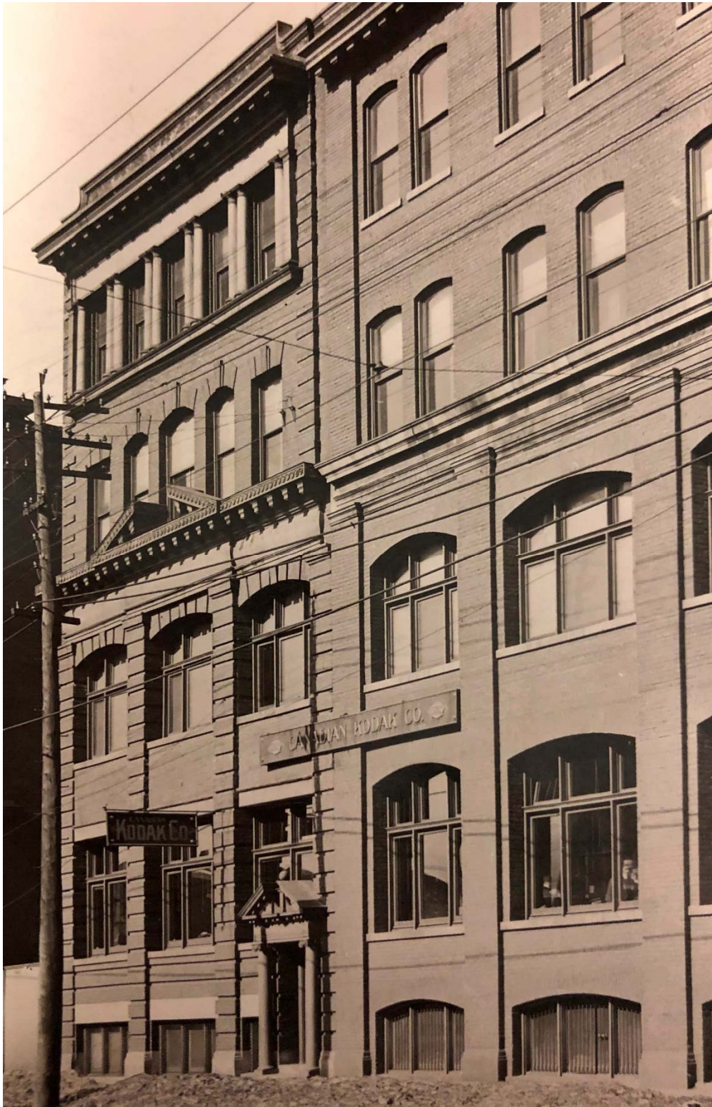
21. 1912 Photograph of 582 King Street West, (detail) showing the details of the original 1902 building with its entrance, the second storey cornice with broken pediment, fourth storey pairs of columns and piers and the Kodak signage (RU)
