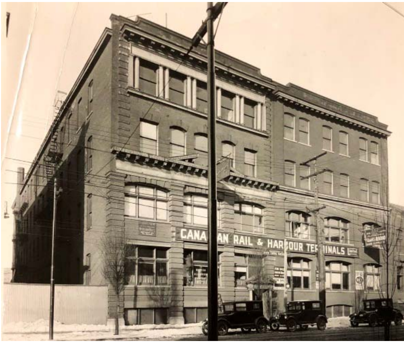
22. 582 King Street West, 1926, during Canadian Rail and Harbour Terminals tenancy (RU)
