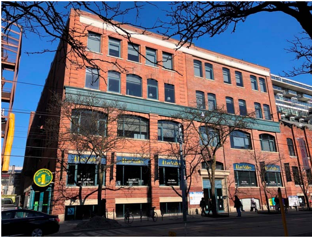
Photograph of the south elevation of the property at 582 King Street West on the north side of King Street West including the two factory-type buildings (Heritage Preservation Services [HPS], 2020)
