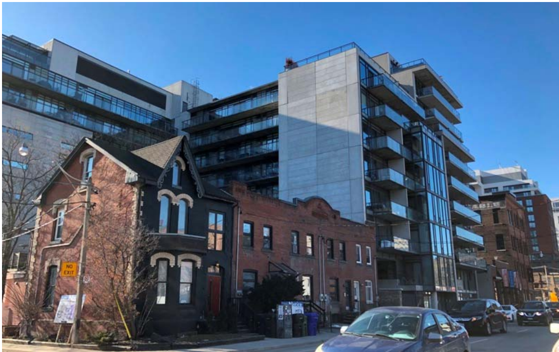
39. Adelaide Street West looking west from 449 Adelaide Street with Victorian houses, recent mid-rise infill and the subject property at 471 Adelaide Street West. (HPS, 2020)
