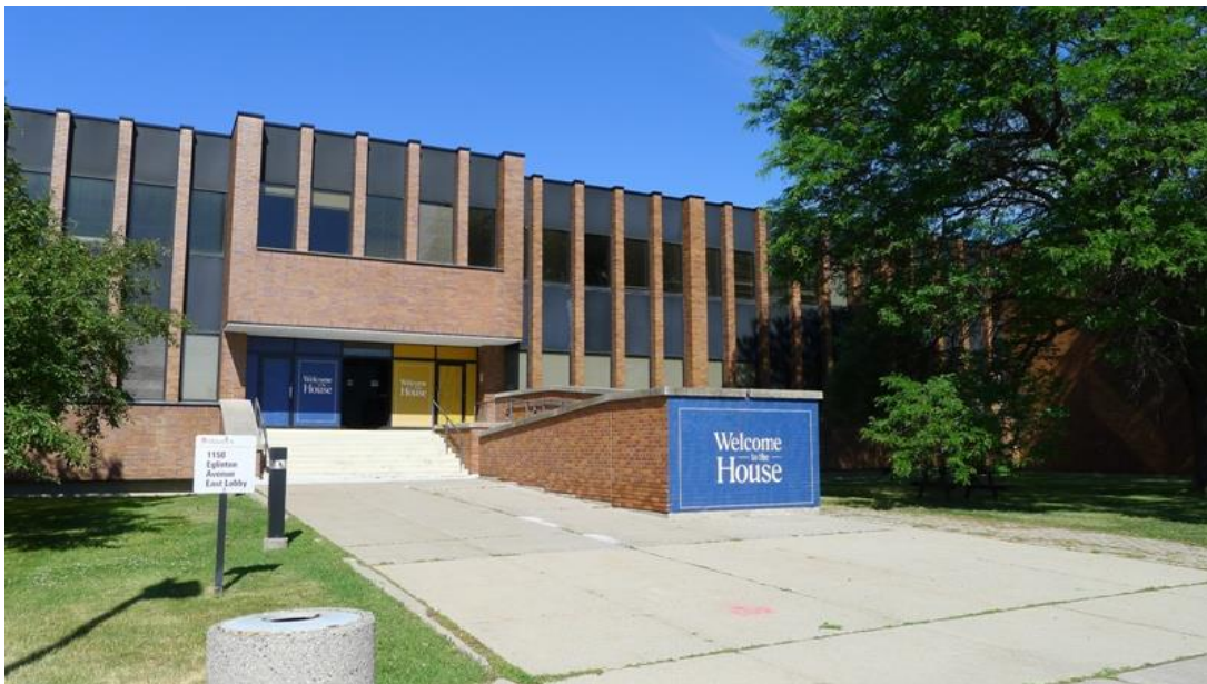
East Entry: showing the same arrangement as the north entry with the broad steps, recessed doors and cantilevered bay here modified with a ramp for universal access. The east elevation faces the parking lot but is set back in lawns with mature trees (HPS, 2016)
