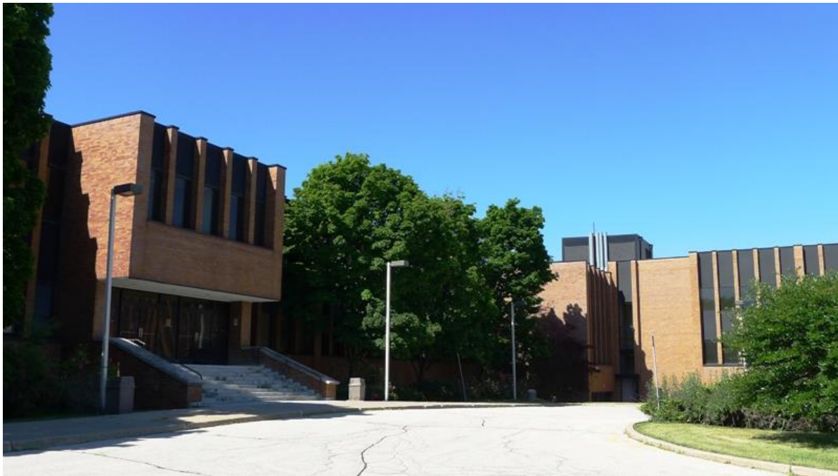
North Courtyard with Main Entry: showing the entry forecourt planting and wide steps leading up to the main entry with a bay cantilevered over the recessed doors (HPS, 2016)
