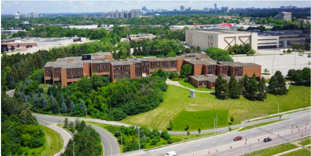
1150 Eglinton Avenue East (Source: Goldsmith Borgal & Company Ltd. Architects, February 13, 2018) - View looking north
