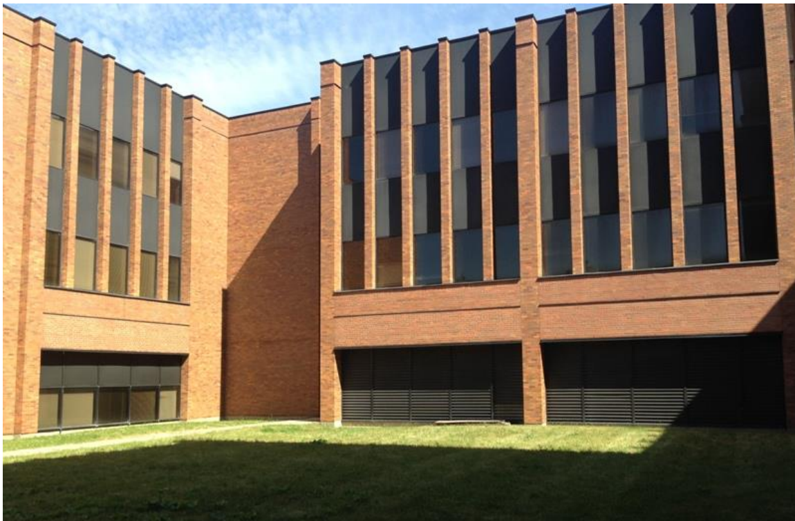
The Former IBM (Canada) Headquarters building: looking north at a south-west-facing courtyard space (HPS, 2016)
