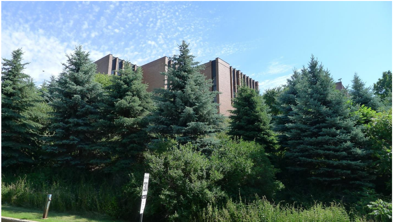
The Former IBM (Canada) Headquarters building: viewed from the driveway from Eglinton Avenue East (HPS, 2016)
