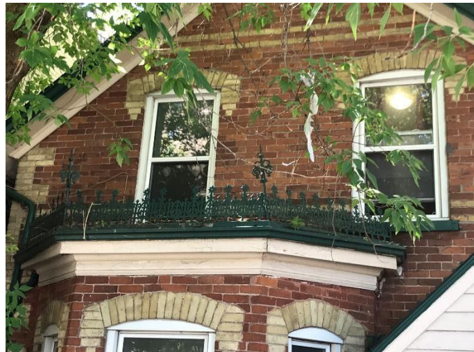
12 and 13. Details of the bay on the east elevation, showing the drop pendant motif headers and saw-tooth soldier course in buff brick below each window opening, as well as the decorative metalwork balustrade crowing the bay window's wooden cornice and flat roof. (HPS, 2018)
