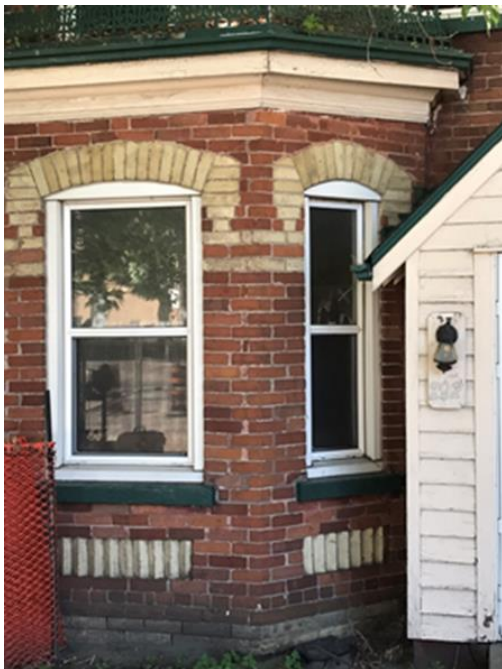
12 and 13. Details of the bay on the east elevation, showing the drop pendant motif headers and saw-tooth soldier course in buff brick below each window opening, as well as the decorative metalwork balustrade crowing the bay window's wooden cornice and flat roof. (HPS, 2018)
