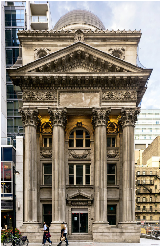
Bank of Toronto Building
