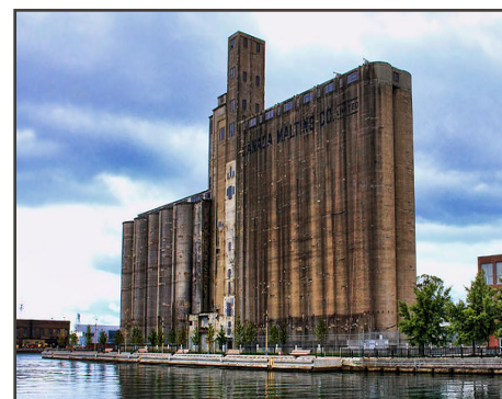
Canada Malting Silos
