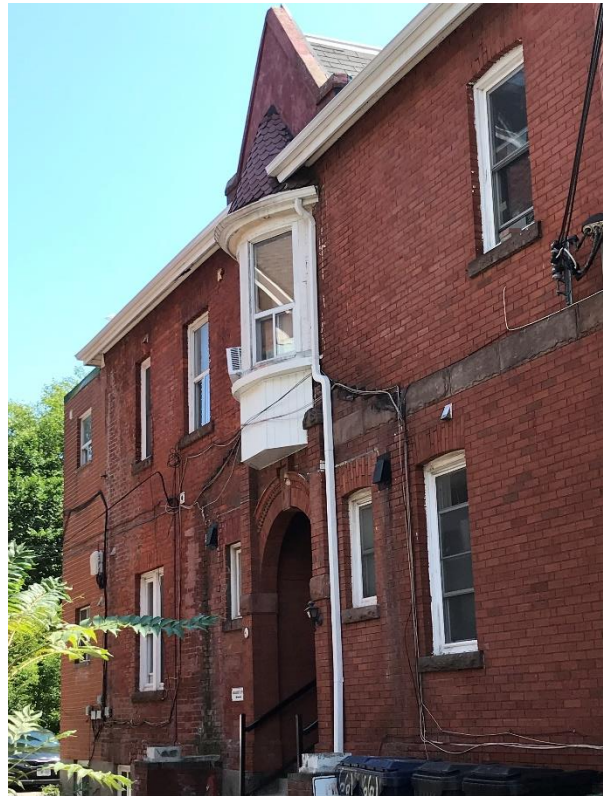
9 and 10: Current photographs showing the 2-storey tower with its rusticated stone cladding at the first floor level, the second storey recessed balcony on the principal (west) elevation (left); at right, the main entrance located on the north elevation. The entry is raised and recessed beyond the red brick, round-arched opening with red sandstone used for the keystone and capitals at the springing joint. (HP, 2020)
