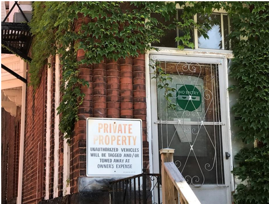
13. Current photograph showing the clustered, terracotta colonettes between the window openings on the principal (west) elevation of the house-form building at 663-665 Huron Street. (HP, 2020)
