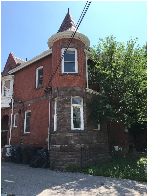
9 and 10: Current photographs showing the 2-storey tower with its rusticated stone cladding at the first floor level, the second storey recessed balcony on the principal (west) elevation (left); at right, the main entrance located on the north elevation. The entry is raised and recessed beyond the red brick, round-arched opening with red sandstone used for the keystone and capitals at the springing joint. (HP, 2020)
