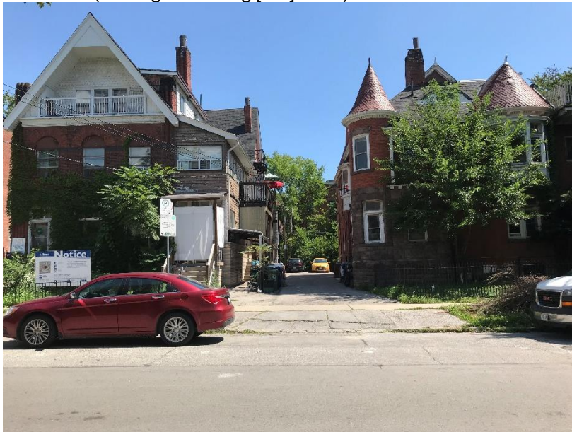
Photo of 663-665 Huron Street at left, and 661 Huron Street at right, including the driveway between the properties that, until recently was covered by a Classically-styled porte-cochere. (Heritage Planning [HP] 2020)
