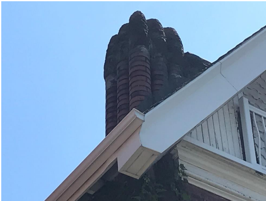
14. The north chimney, which is also composed of terracotta colonettes. (HP, 2020)
