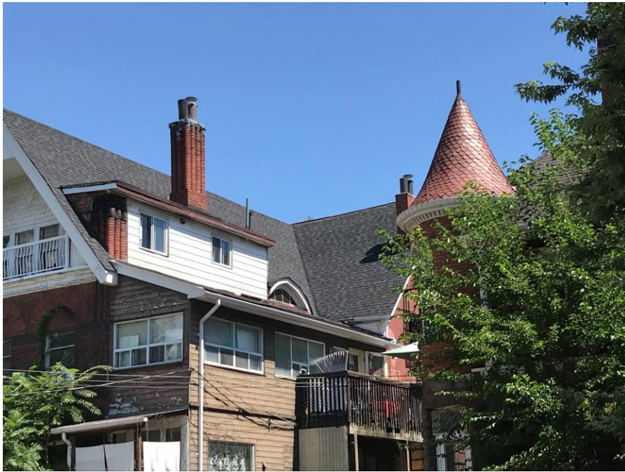
13. Current photograph of 663 Huron Street looking northeast and showing the unique, terracotta colonette clusters supporting the shed dormer roof on the south elevation and the south chimney. (HP, 2020)
