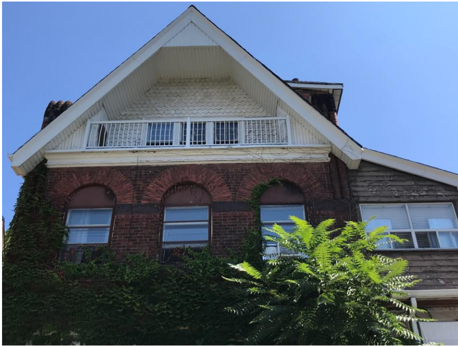
12. The second and third storeys of the principal (west) elevation at 663-665 Huron Street, showing the red brick and sandstone round-arched window openings and inset balcony in the roof gable with its half-cove shingling. (HP, 2020)
