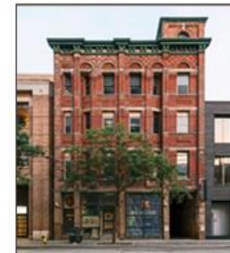
Nealon House, 197 King Street East
