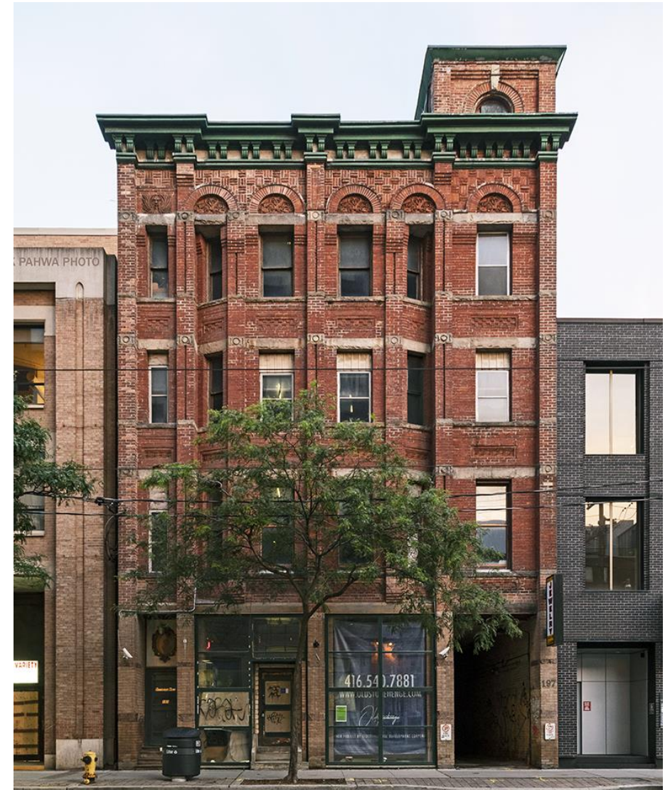
Nealon House, 197 King Street East
