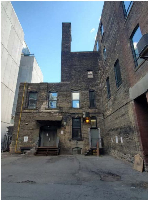
4. Detail of the rear (north) elevation of 578 King Street West, which can only be accessed from a laneway entrance from Portland Street (Heritage Planning Image, 2020)
