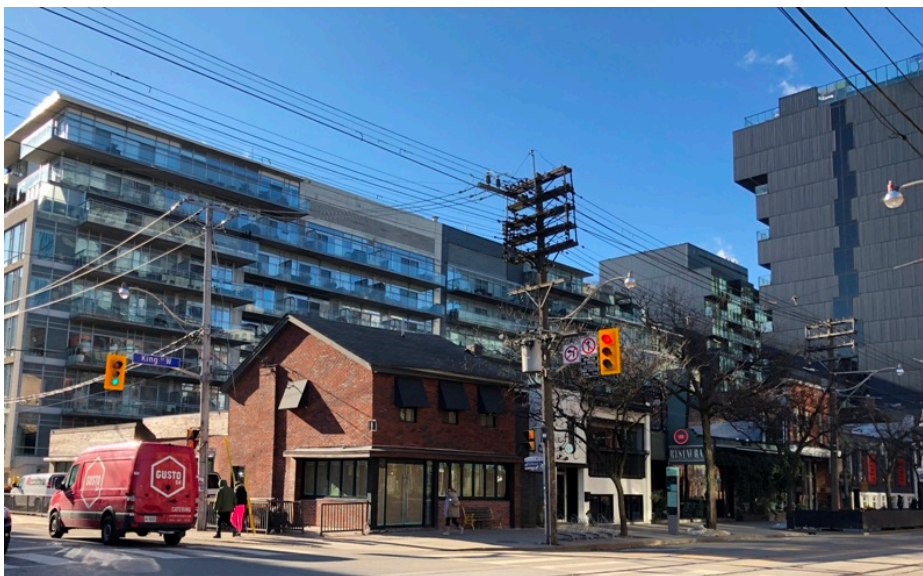
18. Southwest corner of King and Portland streets, c.1870s house-form building (Heritage Planning Image, 2020)
