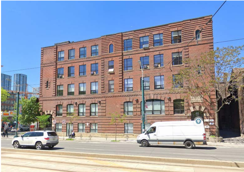
15. Business Systems Limited Warehouse (1907) at 46 Spadina Avenue, Burke and Horwood (Google Street View, 2019)
