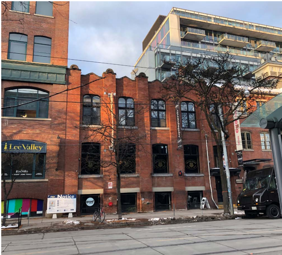
1. Detail of the principal (south) elevation of 578 King Street West (Heritage Planning Image, 2019)
