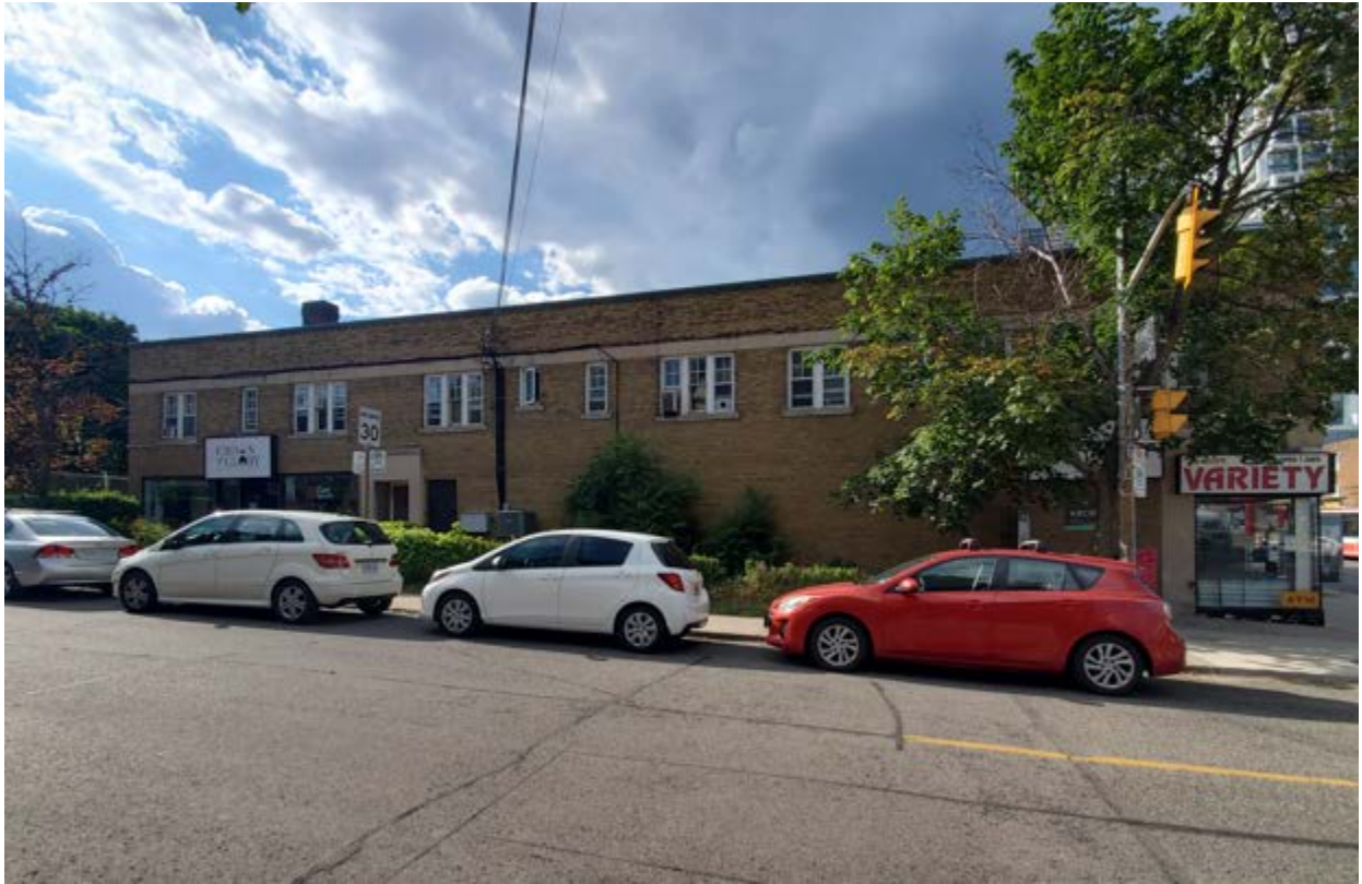
10. Side (south) elevation along Manor Road West of the property at 2100 Yonge Street (Heritage Planning [HP] Photo)
