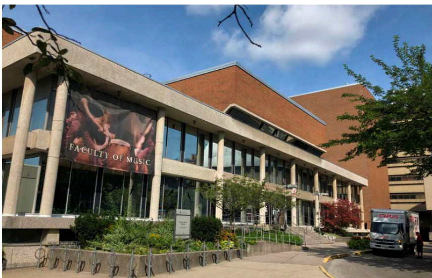
40. Edward Johnson Building, principal (east) elevation showing the two storey colonnade, the brick attic originally designed for the library and to the right, the fly tower of MacMillan Hall. (HP, 2020)
