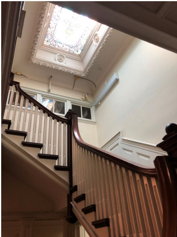
36 and 37. Grand Staircase, upper levels with the finely crafted handrails and newel posts and balusters, wood panelling and stained-glass skylight (HP, 2020)
