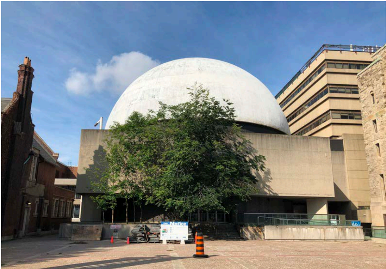
56. McLaughlin Planetarium, principal east elevation facing Queen's Park with Falconer Hall at the left and the ROM to the right (HP, 2020)
