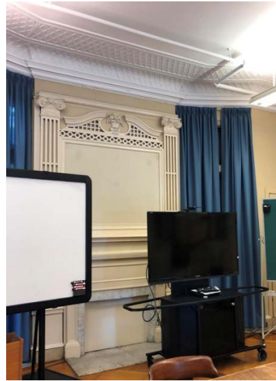
34 and 35. Solarium (also referred to as the music room) added in 1914 with marble stairs, wrought iron handrails, and plaster ceiling, cornice and fireplace decoration featuring trellis, and floral motifs (HP, 2020)
