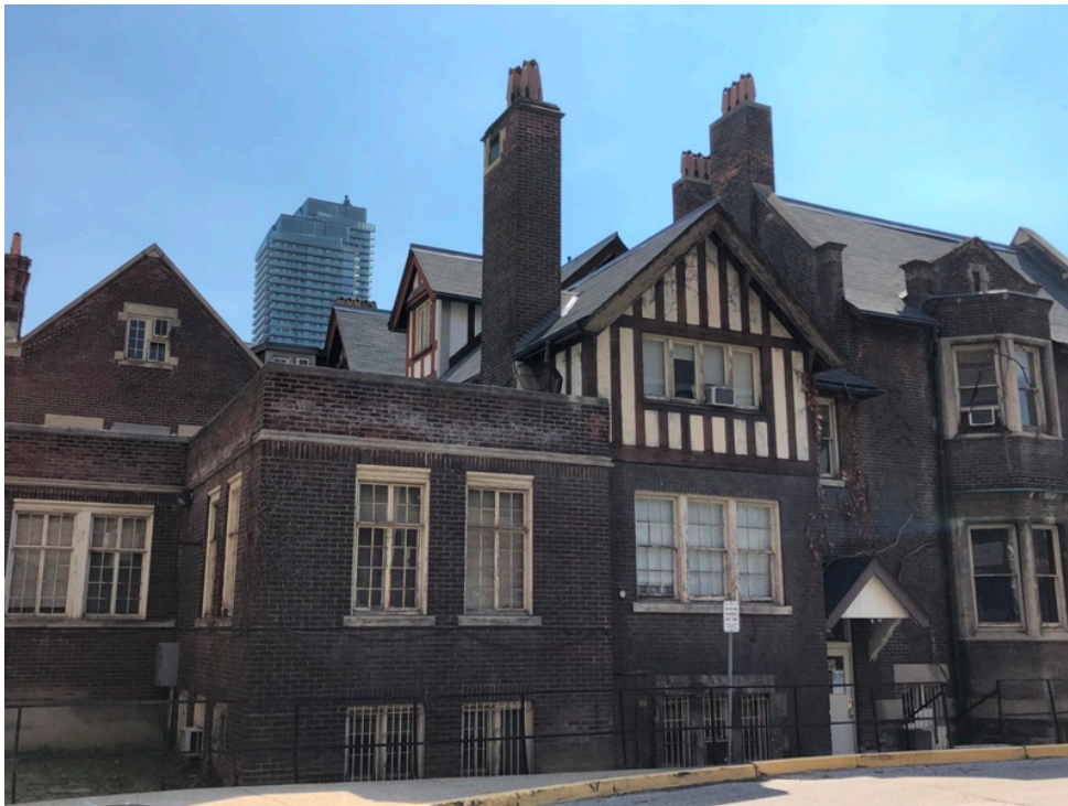
22. West facade showing the post-1925 basement and first floor addition on the left (HP, 2020)
