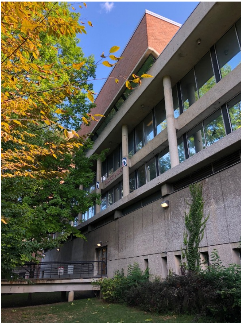
45. EJB West elevation with lower entrance and bridge connecting with Philosopher's Walk (HP, 2020)
