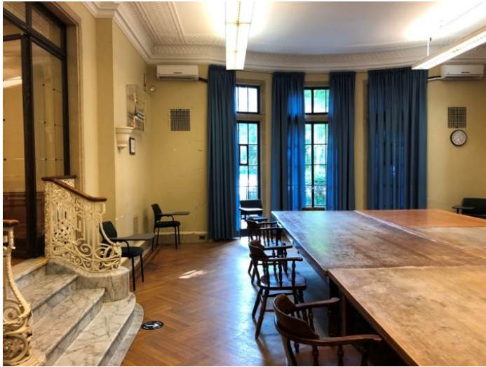
34 and 35. Solarium (also referred to as the music room) added in 1914 with marble stairs, wrought iron handrails, and plaster ceiling, cornice and fireplace decoration featuring trellis, and floral motifs (HP, 2020)
