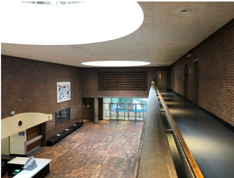
52. EJB, main entry foyer at the balcony level with its palette of brick, brick screens concrete columns, lintels and handrails and glazed variegated brown tiles. To the left the ivory coloured, flattened, curved pediment indicates the corridor leading to the Rupert E. Edwards library (HP, 2020)
