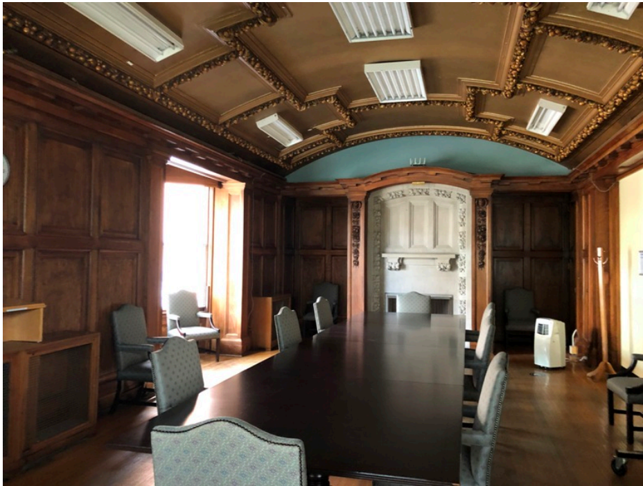
32. Billiard Room (1908 addition) with Circassian walnut panelling and stone fireplace
