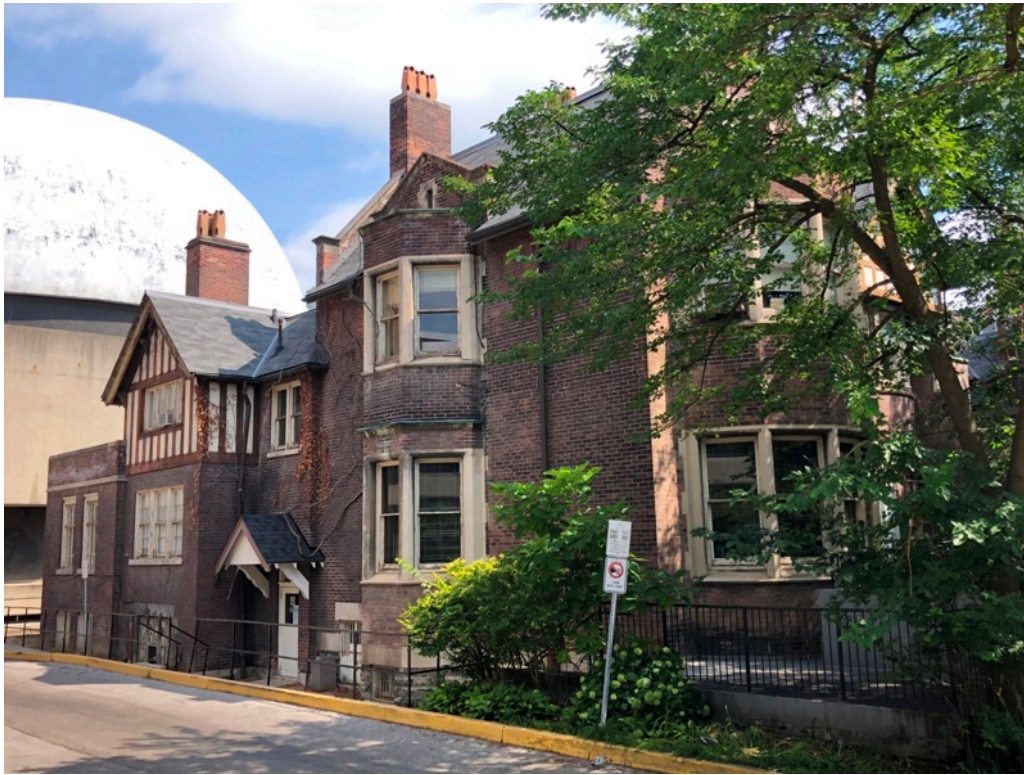
21. Corner of the south and west facades showing the 1908 with the two projecting bay windows, and the later kitchen wing with its half timbering on the upper level. To the left of the wing is a post-1925 addition which accommodated dining facilities (HP, 2020)
