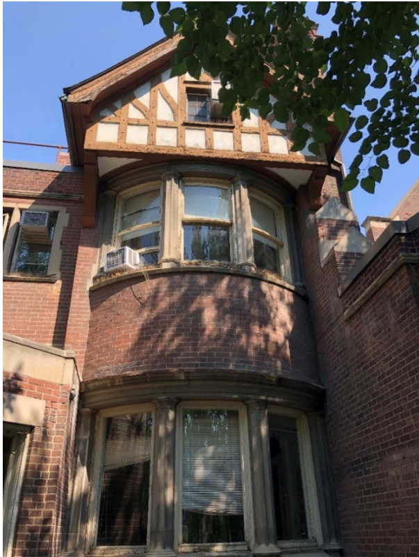
19. South facade showing the original bay window of the former Palm Room between the solarium extension and the later addition of an exit door. Note the Elizabethan detailing of the engaged columns flanking the window openings (HP, 2020)
