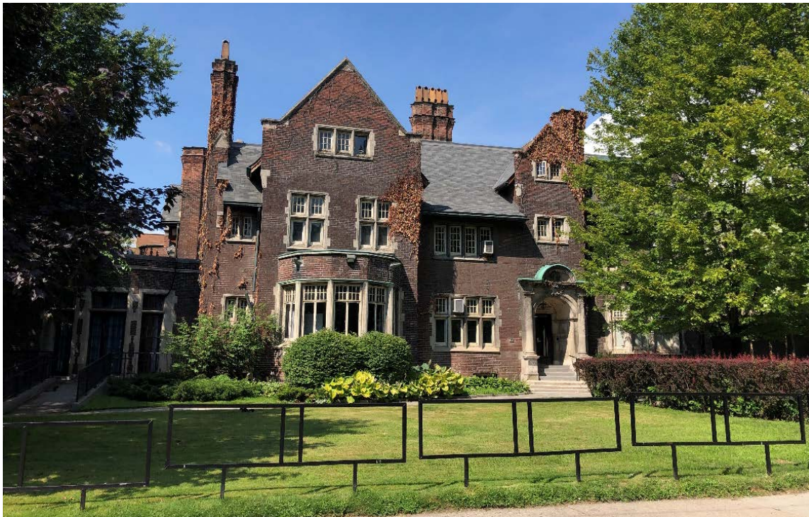
16. Wymilwood/Falconer Hall, principal east elevation facing Queen's Park (Heritage Planning [HP], 2020)
