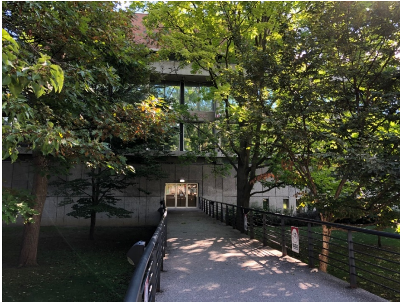
46. Pedestrian bridge leading from Philosophers Walk to the lower levels of the EJB (HP, 2020)
