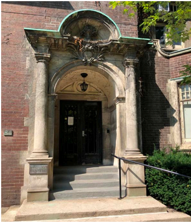
18. Wymilwood, east facade, stone door case and recessed entrance (HP, 2020)
