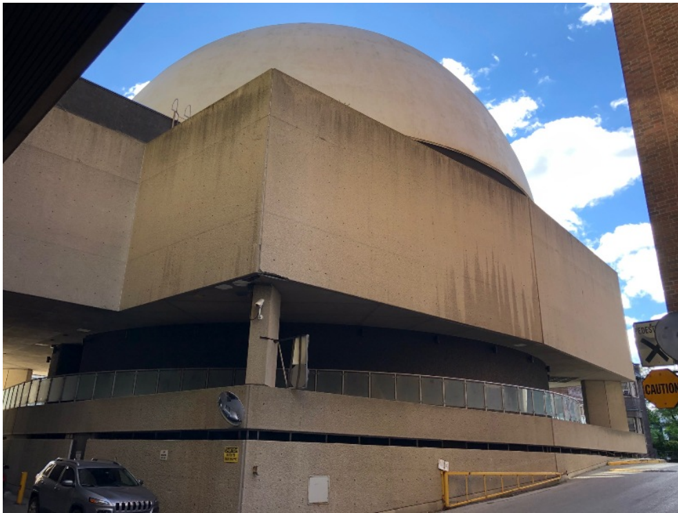
58. McLaughlin Planetarium, west and north elevations (HP, 2020)
