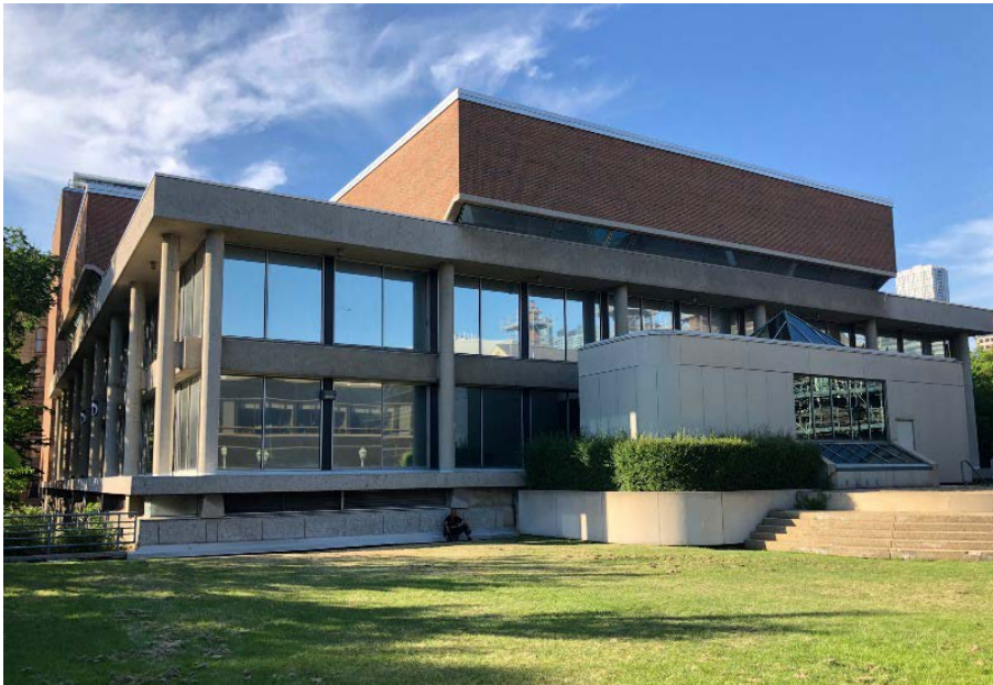
41. Edward Johnson Building, south elevation showing the 1988 addition of the stairs and entry to the Rupert R. Edwards wing containing a two-storey underground library under the lawn (HP, 2020)
