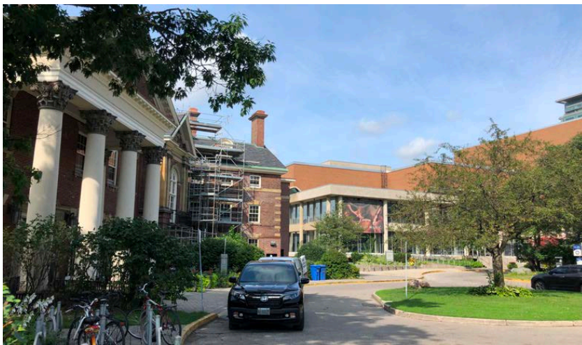
39. View of the Edward Johnson Building (right), south-east corner, as approached from Queen's Park and Flavelle House with its columned entrance portico (left) (HP, 2020)
