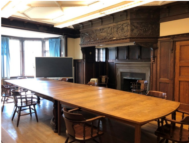
27. Living Room with Elizabethan fireplace with an inglenook, and Elizabethan-style ornament on the ceilings and wood panelling and cornice (HP, 2020)
