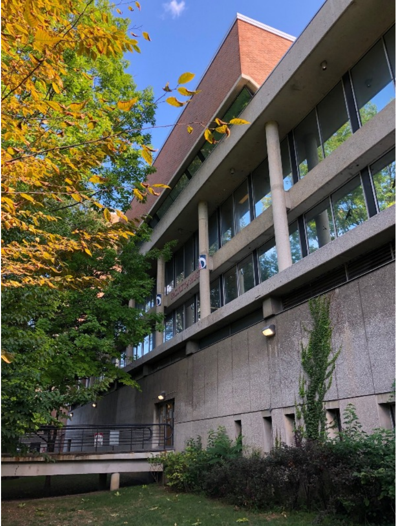
45. EJB West elevation with lower entrance and bridge connecting with Philosopher's Walk (HP, 2020)
