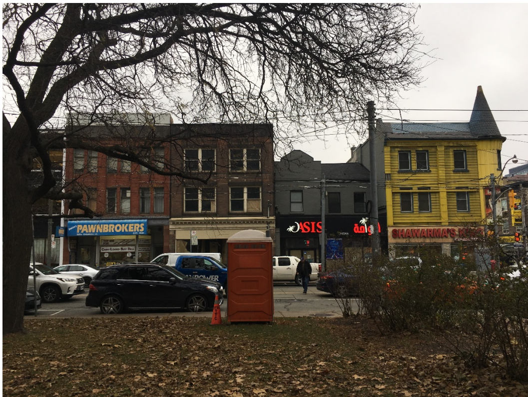
Existing condition of 60 Queen St. East and 131, 133 and 135 Church St.
