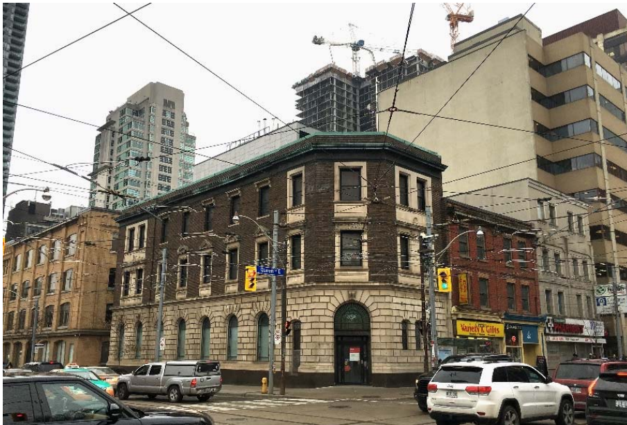
Adjacent listed property at 79 Queen Street East (Former Bank of Nova Scotia)
