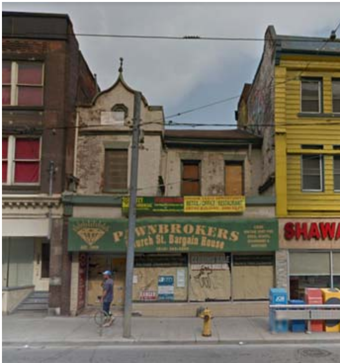
4f. 131 Church Street, showing the original ogee-arched parapet containing an octagonal window opening, 2015
