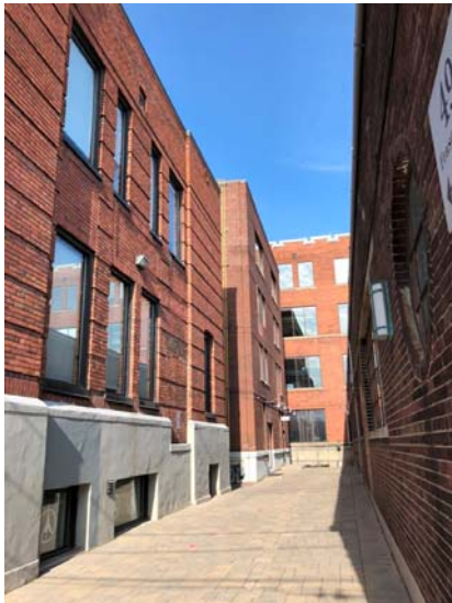
43. View (left) of the south elevations of 47 and 49 Fraser Avenue along a passageway terminated by 53 Fraser Avenue. Note the bilateral symmetry of the projecting outer bays, the pattern of striated brick work creating piers between windows with decorative panels beneath the windows on 47 Fraser Avenue (HP, 2020)
