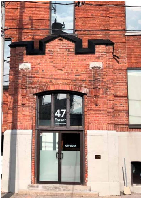
40. Projecting Entry Porch at 47 Fraser Avenue with the shield motif above the door, flanked by two pinnacles and with the crenellated roof line (HP, 2020)
