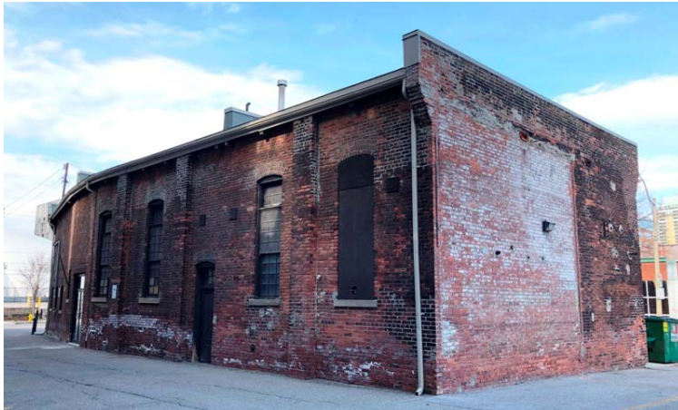
37. South-west elevation of the powerhouse showing the double-height triple sash windows flanked by brick piers with brick corbels on the end wall (HP, 2020)
