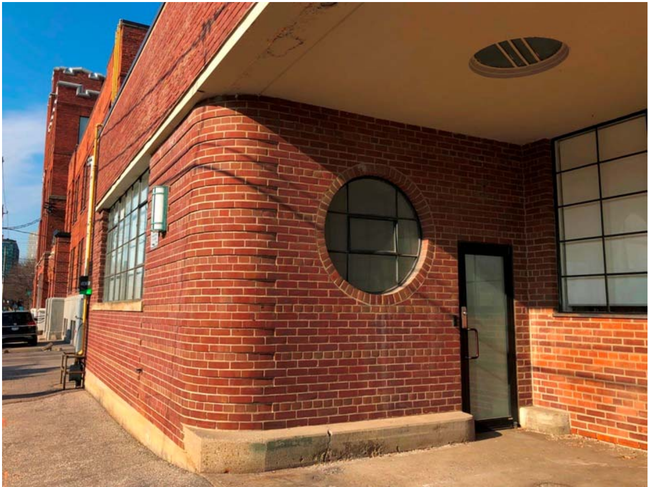
48. Photograph of the Entrance at 41 Fraser Avenue showing the details including the recessed brick banding, the bull's eye window, the light fitting recessed in the ceiling. The window at the right and the wall beneath it are later alterations closing off the original garage entry. (HP, 2020)
