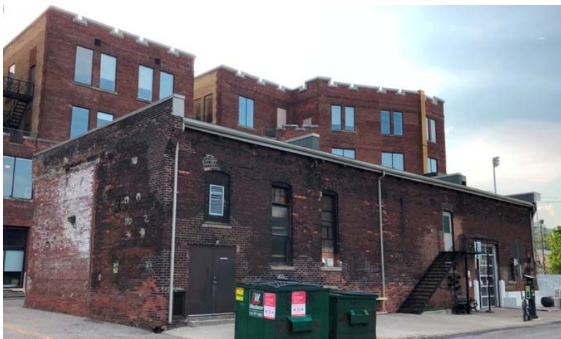
38. South and East elevations of the powerhouse showing alterations with new doors and altered window openings (HP, 2020)
