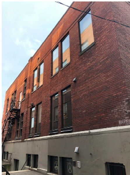
43. View (left) of the south elevations of 47 and 49 Fraser Avenue along a passageway terminated by 53 Fraser Avenue. Note the bilateral symmetry of the projecting outer bays, the pattern of striated brick work creating piers between windows with decorative panels beneath the windows on 47 Fraser Avenue (HP, 2020)
