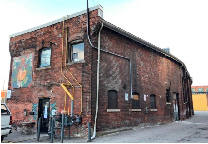
36. North and west elevation of the powerhouse showing the angled wall which was altered to accommodate the railway spur (HP, 2020)
