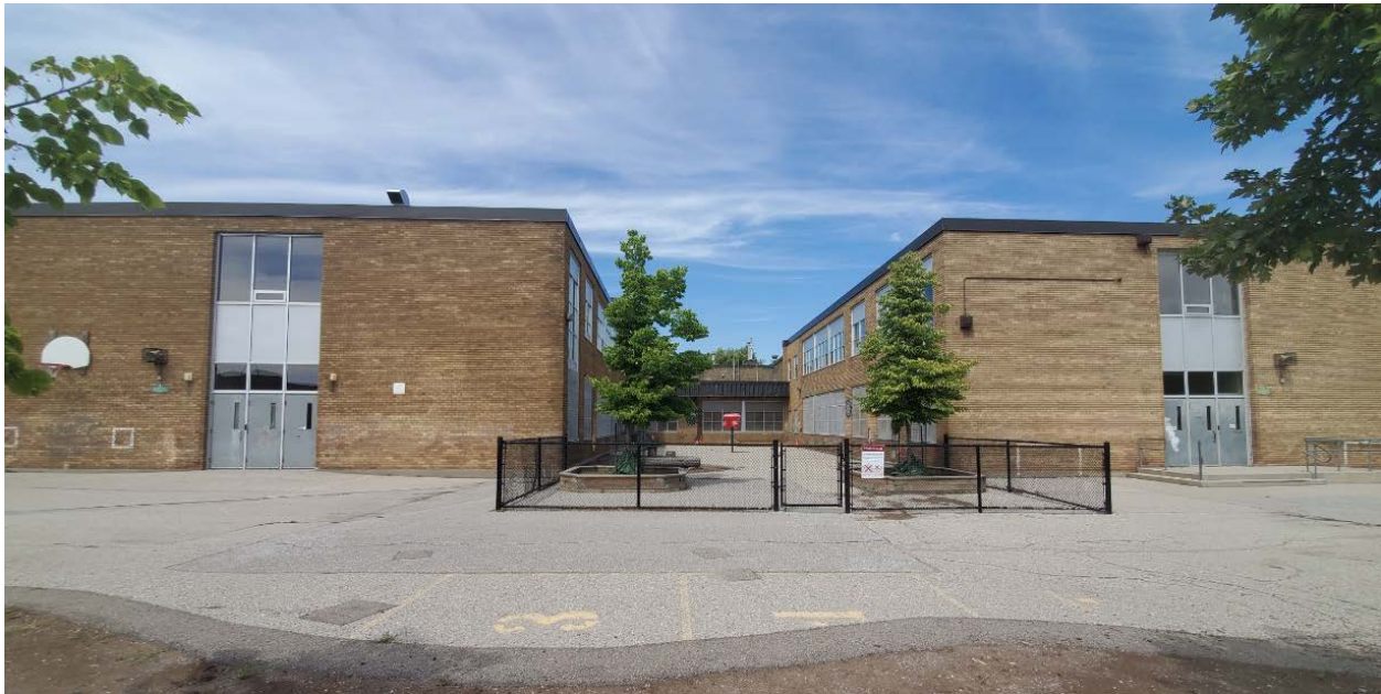
Detail of the rear (south) elevation of St Leo's Catholic School, showing the 1963 addition (left) and 1958 addition (right) (Heritage Planning Image, 2020)
