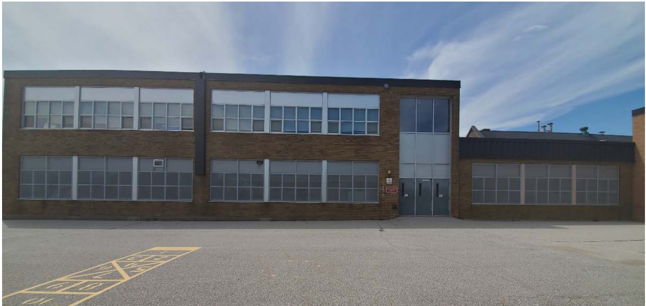
Detail of the side (east) elevation, showing the 1963 addition (left) and the 1956-7 (right) (Heritage Planning Image, 2020)
