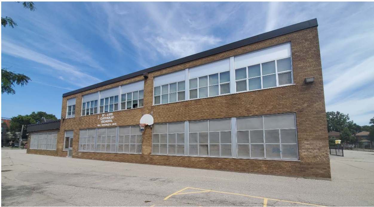
Detail of the side (west) elevation of St Leo's Catholic School, showing the 1956-7 addition (left) and 1963 addition (right) (Heritage Planning Image, 2020)
