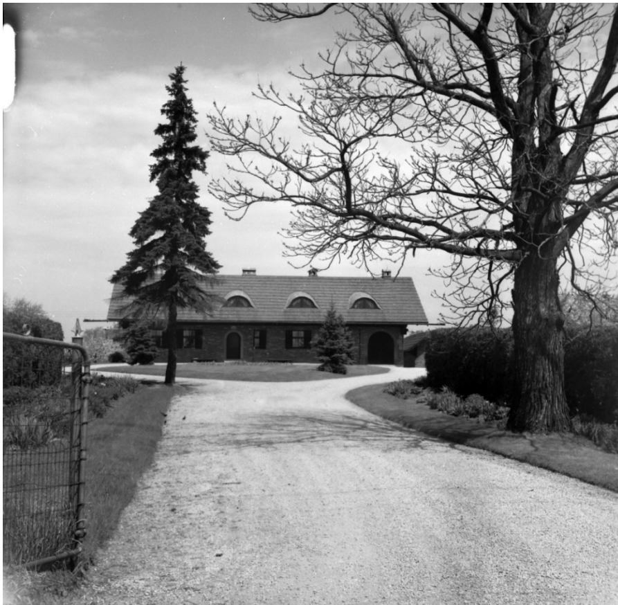
6. Frederic J. A. Davidson's 'Brookwood' built after 1911 on the east side of Royal York Road and backing onto Mimico Creek. Like Davidson's later houses at 96-98 Superior Avenue and 214 Queens Avenue, 'Brookwood' displays a cedar shingle gable roof and 1.5-storey block plan dwelling constructed of stone that was also likely locally sourced from Mimico Creek. (Toronto Public Library, 1955).
