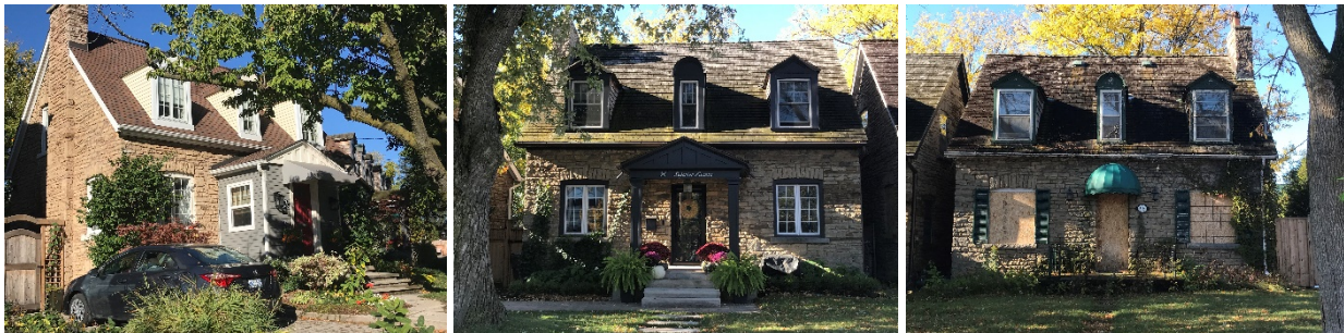
[Left to right]: Photos of the properties at 214 Queens Avenue, 96 and 98 Superior Avenue showing the principal (east) elevations (Heritage Planning [HP] 2020)
