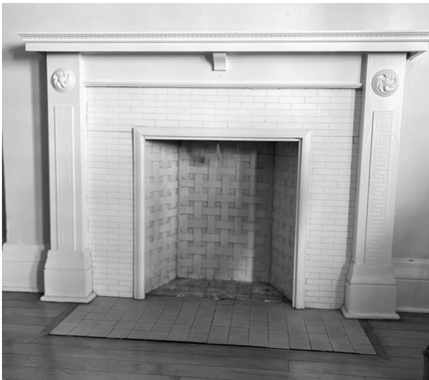
40. Typical fireplace with mantel and ceramic brick tiles provided by the Hawes' brothers as per architect's specifications. Note the basket weave of the ceramic firebox (HP, 2020)
