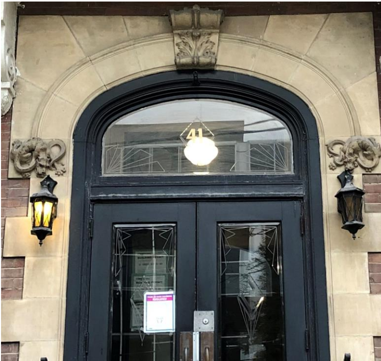
22. Photograph showing the carved stone elements of the door case, the keystone with acanthus leaf moulding and the dragons on the impost blocks and the etched glass details of the transom with the entrance numbers and the 'S' and 'G' on the pair of doors (partly obscured by temporary signage) (HP, 2020)
