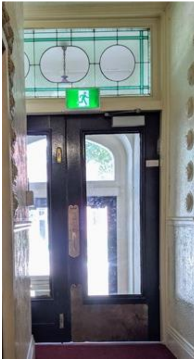
28 and 29. Entrance lobby with the elevator on the left and the pair of oak doors with the green stained glass transom light as designed and specified by A. R. Denison. The architect also specified the four-foot dado seen on the left. (HP, 2019)
