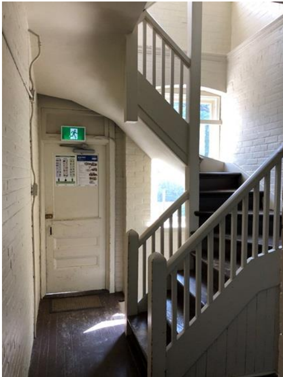
34. and 35. Rear service stairs showing the wood handrails and treads and the internal brick work now painted (HP, 2019)
