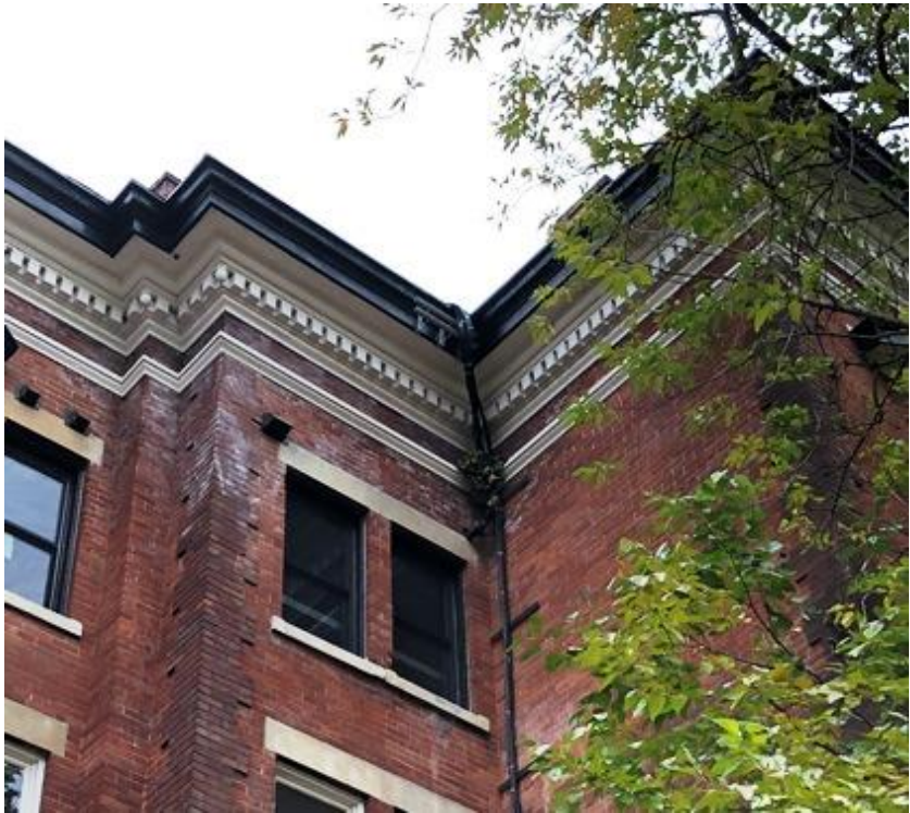
25. Photograph of the cornice detail on the north elevation (HP, 2020)
