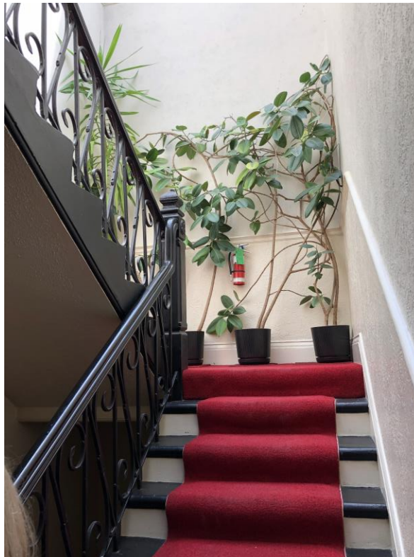
30 and 31. Stair case of wrought iron with cast iron newel posts and cherry hand rail as specified by A. R. Denison. (HP, 2019)
