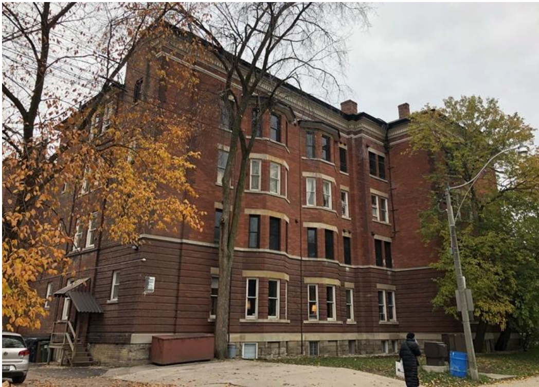
Spadina Gardens, 41 Spadina Road, north elevation facing Lowther Avenue and rear east elevation (HP, 2020)
