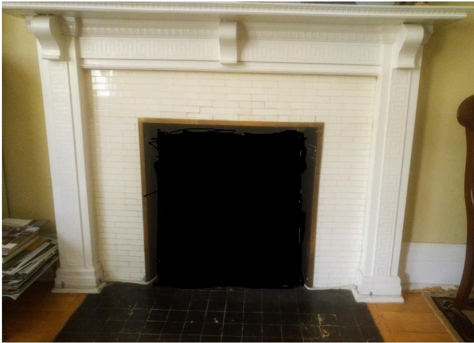
41. One of the apartment fireplaces showing the surround with the Greek key motif, the console bracket and mouldings, cream coloured glazed brick tiles, black square floor tiles (HP, 2020)
