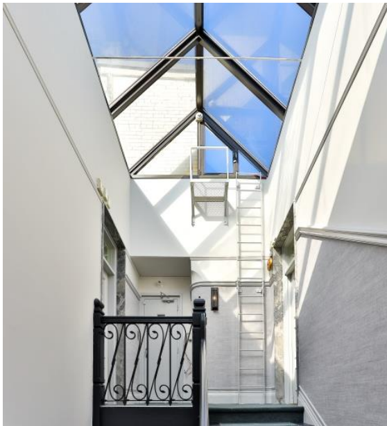
32. Skylight at the top of the stairs and original cast and wrought iron handrails (41-45 Spadina Road Property Inc., 2020)
