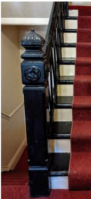
30 and 31. Stair case of wrought iron with cast iron newel posts and cherry hand rail as specified by A. R. Denison. (HP, 2019)
