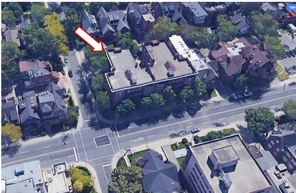
2. Aerial view of the property at 41 Spadina Road. (Google Maps, 2020)
