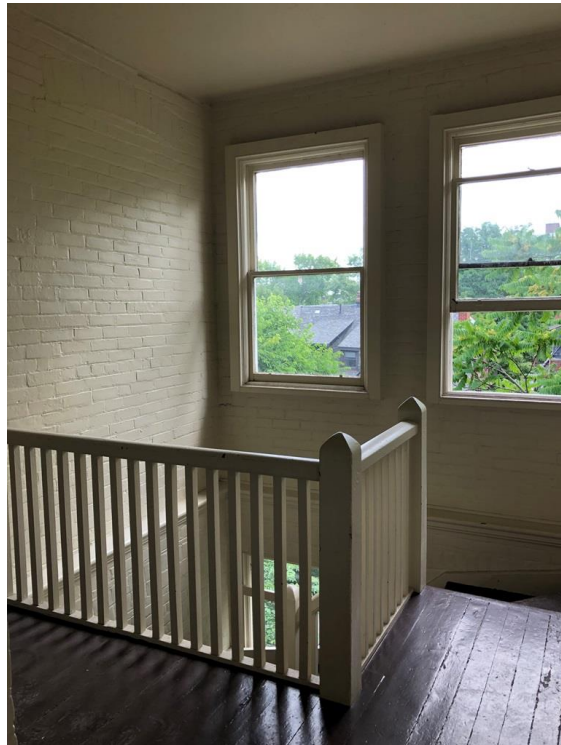
34. and 35. Rear service stairs showing the wood handrails and treads and the internal brick work now painted (HP, 2019)
