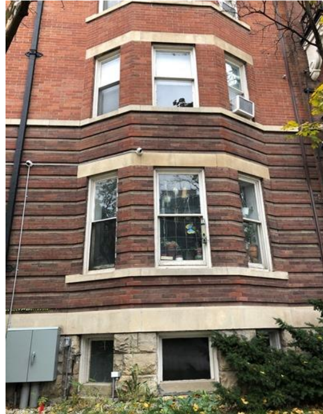
Photograph of one of the bay windows on the west elevation showing the materials including the rough-hewn stone blocks, Roman stone bands and lintels, purple bricks of the rusticated base and the red brick of the upper stories
