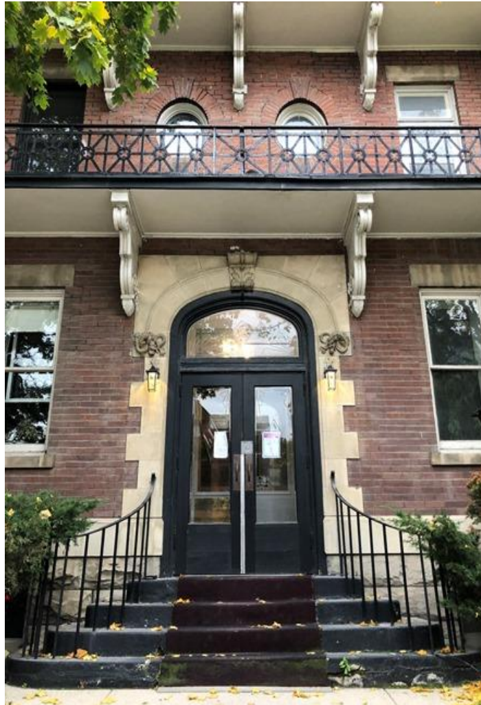
Principal entrance bay at 41 Spadina Road
