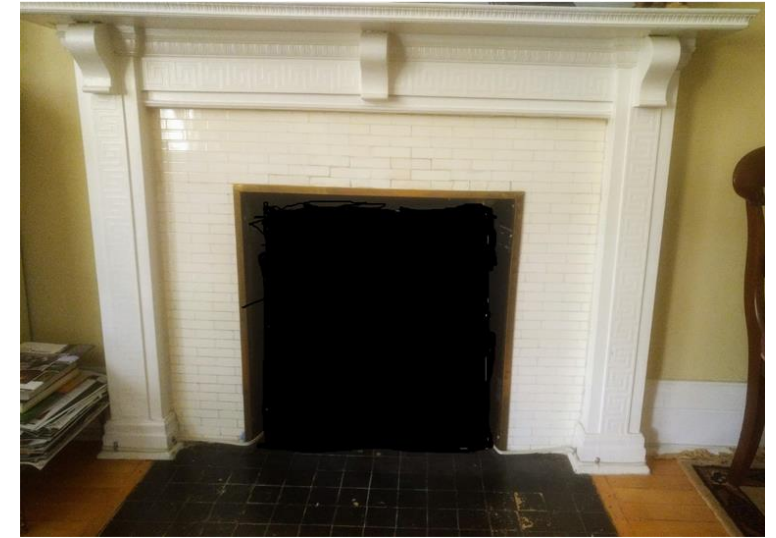
Photographs showing original door hardware (top) and one of the original fireplaces with glazed tile surround and mantel piece (bottom)
