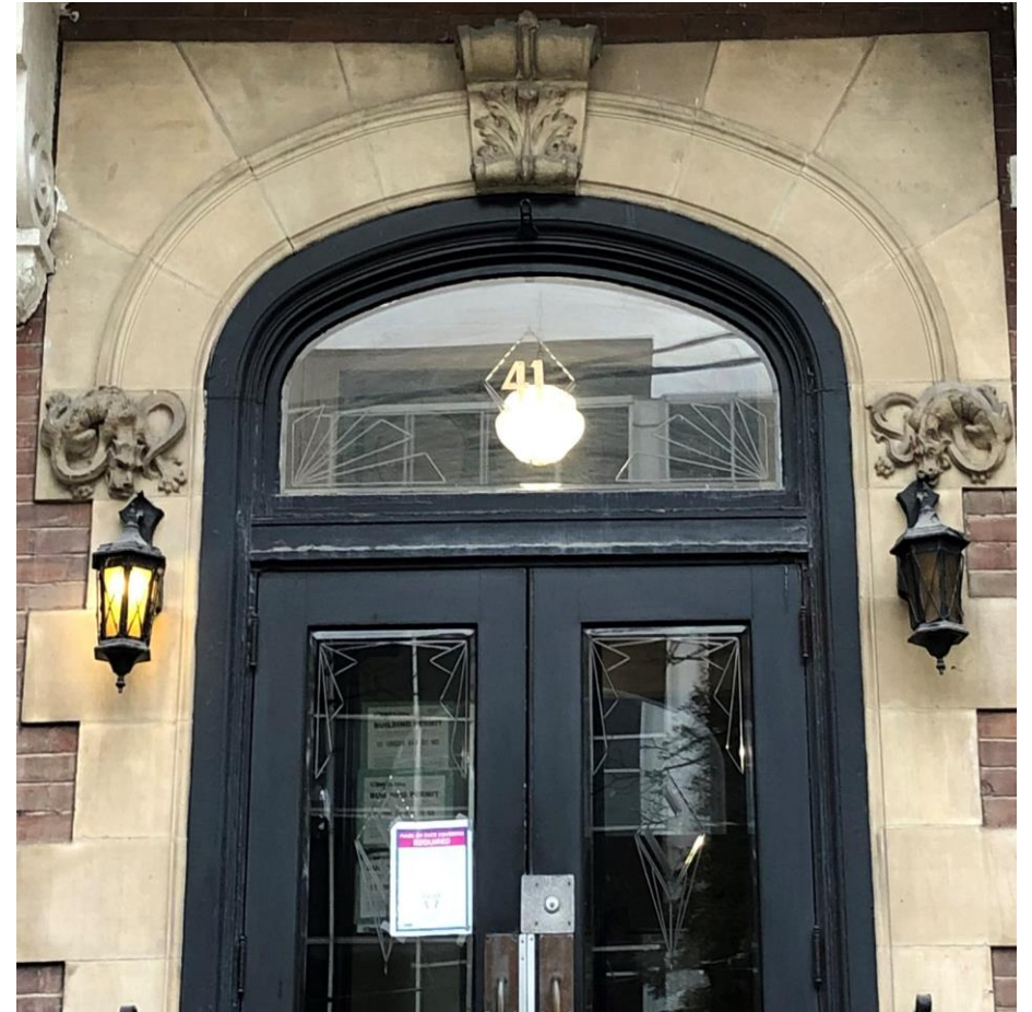
Photograph showing the carved stone elements of the door case, the keystone with acanthus leaf moulding and the dragons on the impost blocks and the etched glass details of the transom with the entrance numbers and the 'S' and 'G' on the pair of doors (partly obscured by temporary signage)
