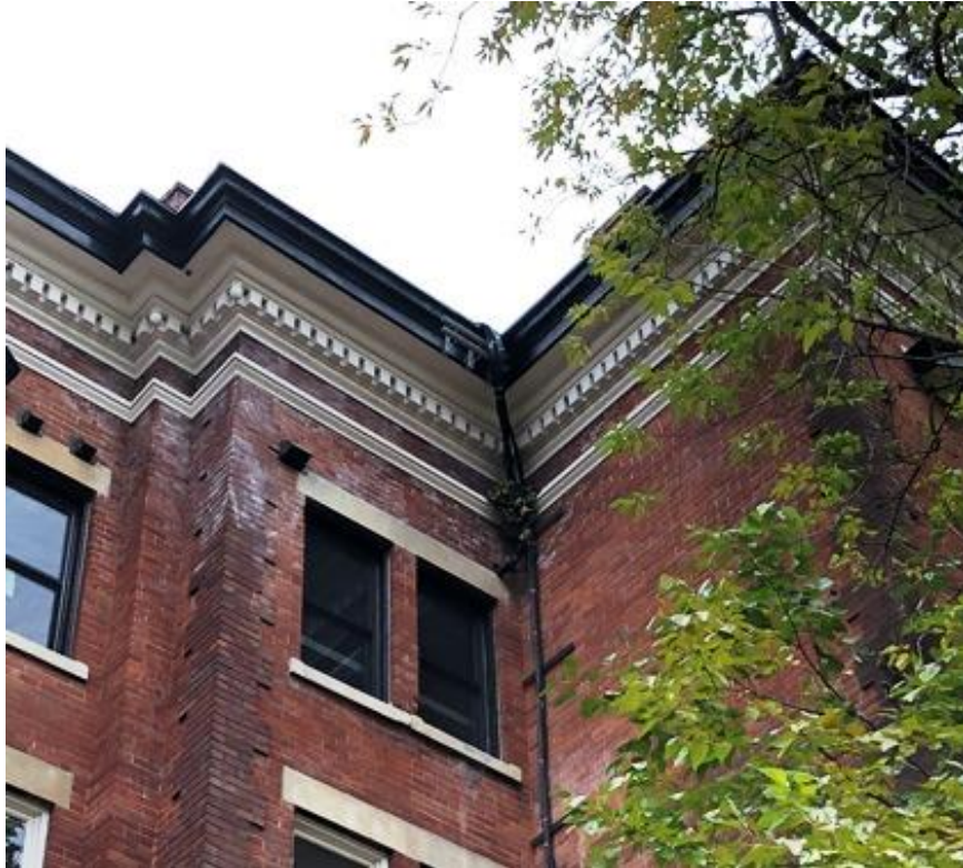
Photograph of the cornice detail on the north elevation
