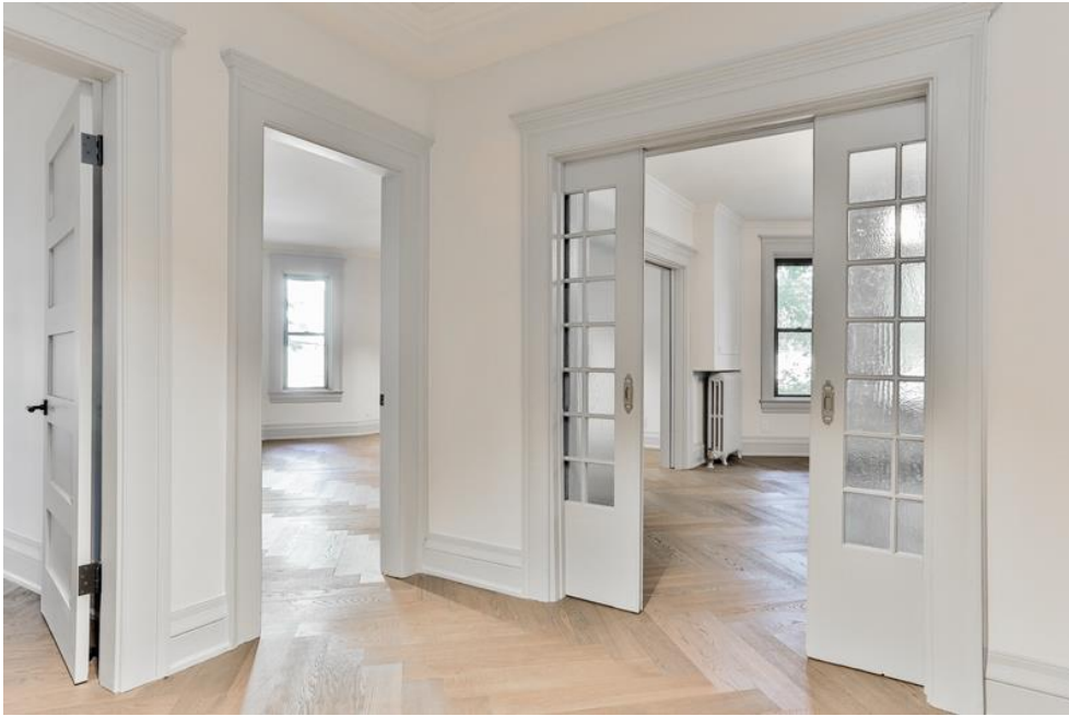
View of a typical apartment from the entrance hall to the den, 'parlor' and dining room showing the pocket doors open between hall and dining room and between the parlor and dining room
