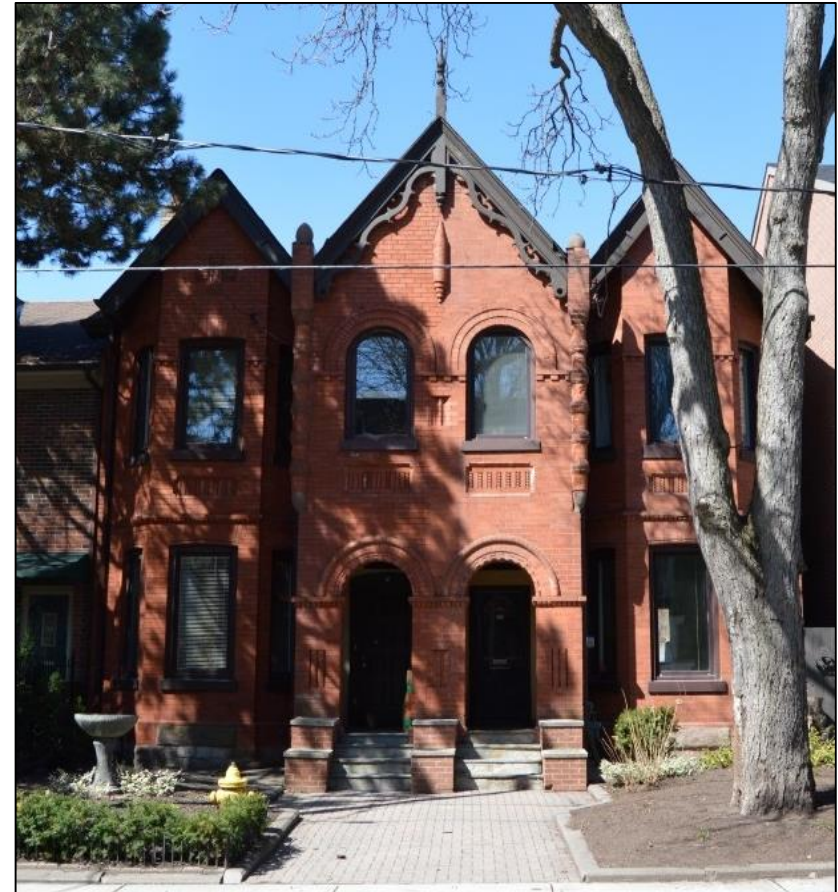
210-212 Berkeley Street, pre-1870 Semi-detached building type Romanesque Revival style
