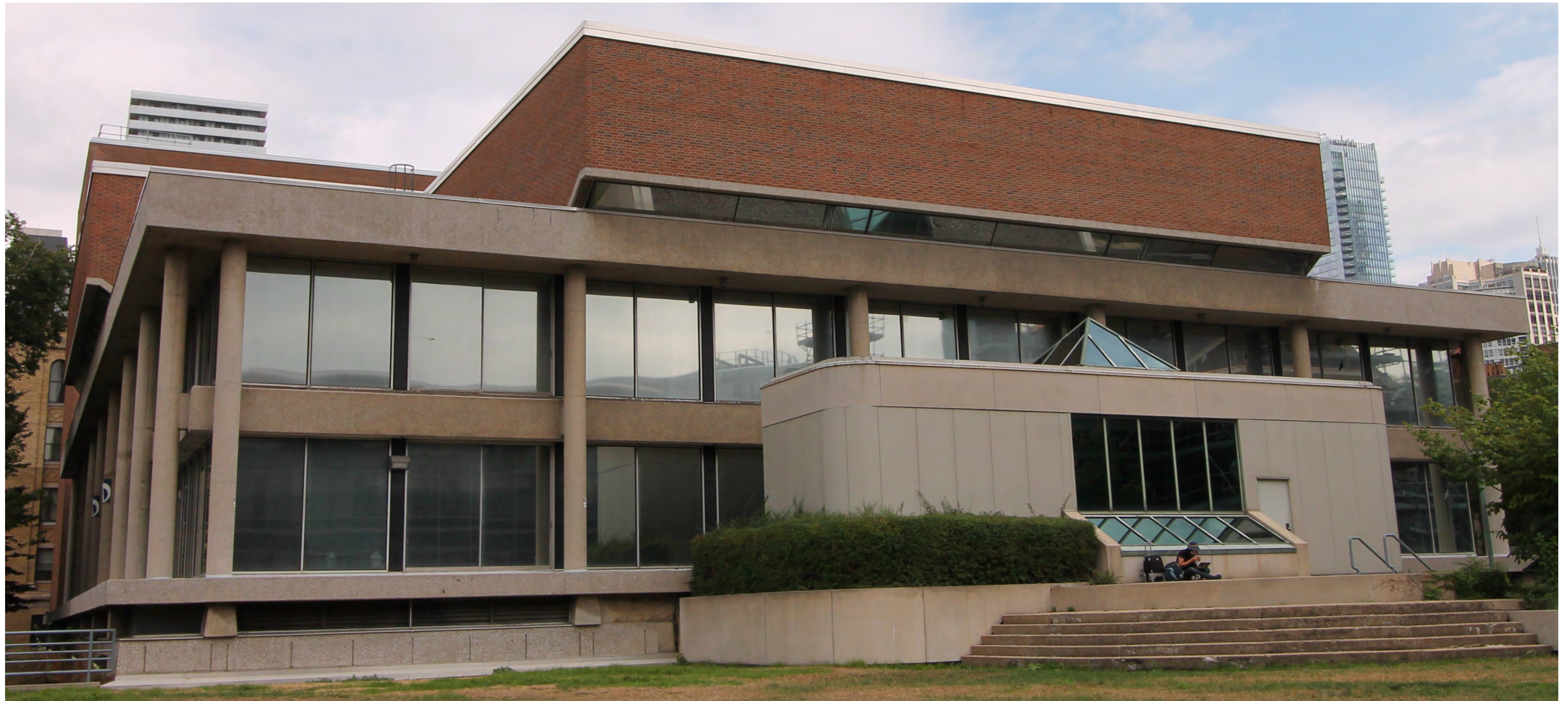
Edward Johnson Building
