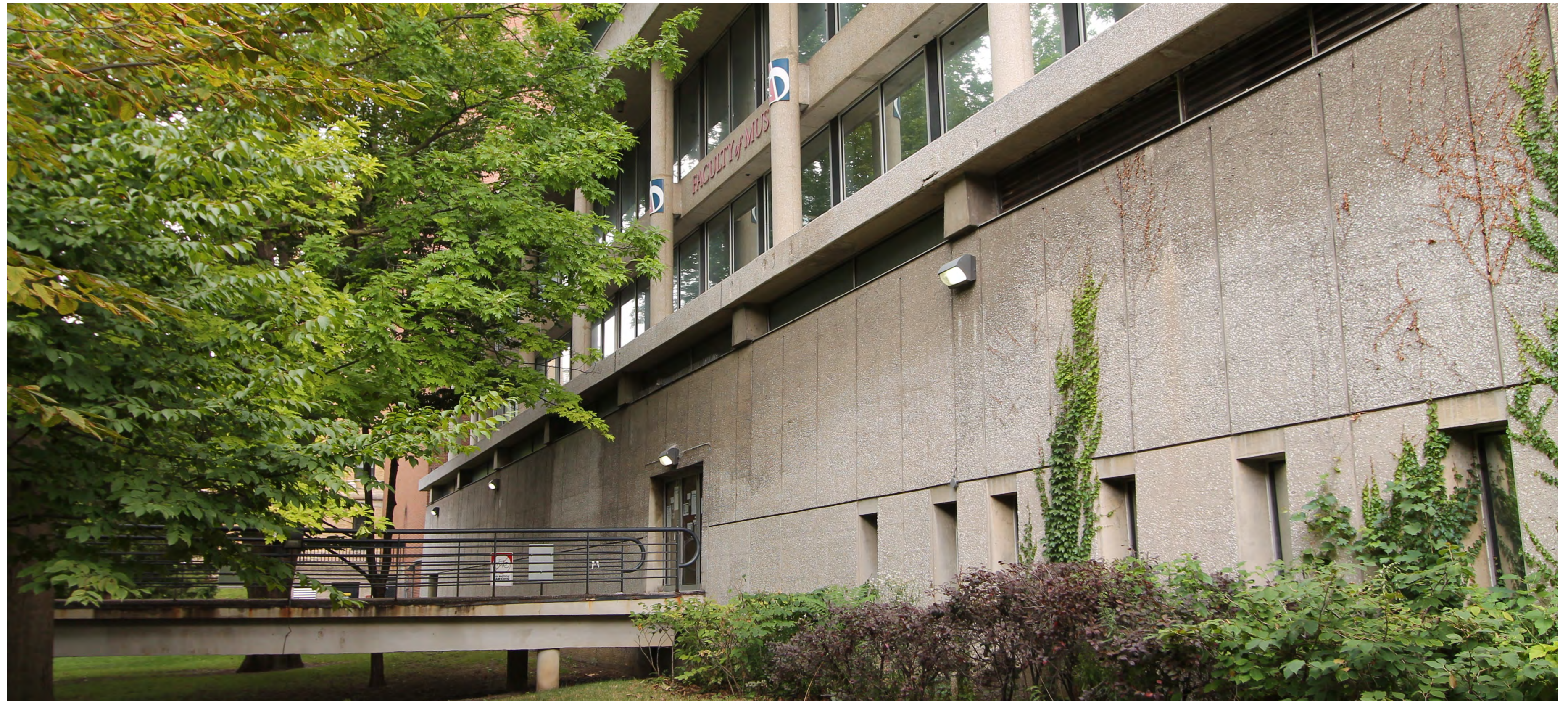
Edward Johnson Building
