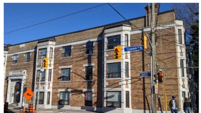
PARC acquired a 39 unit rental building with the support of the City and the Province. 2020.
