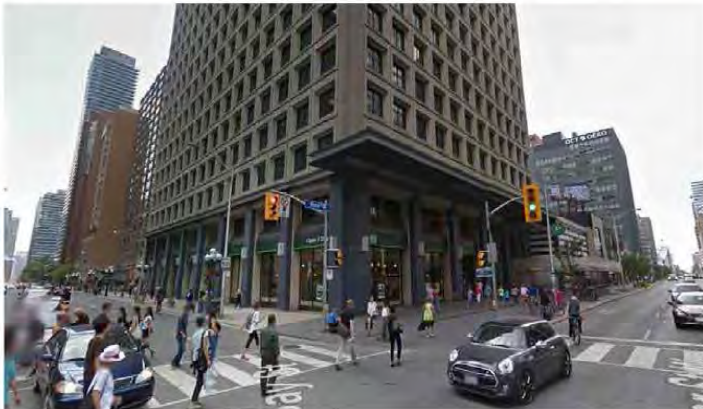
Bay and Bloor South West Corner
