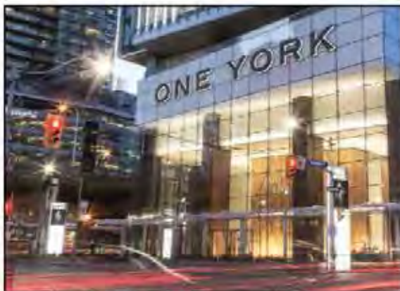
Figure 8.13: Sweeny & Co Architects and KDA
