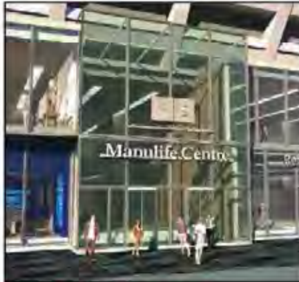
Figure 1.1: Bloor Street Entrance
