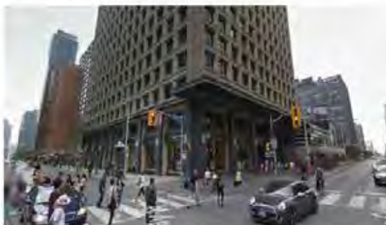
Bay and Bloor South West Corner
