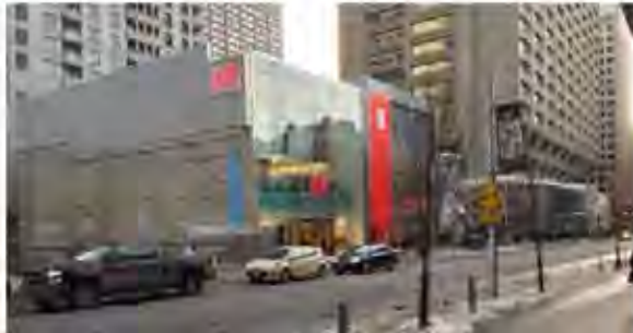
Scotiabank and H&M Branding at 4 th Floor Level - Southeast
