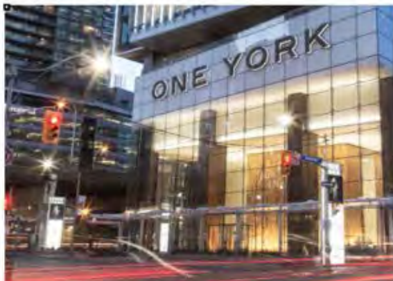
Figure 8.14: Sweeny & Co Architects and KDA
