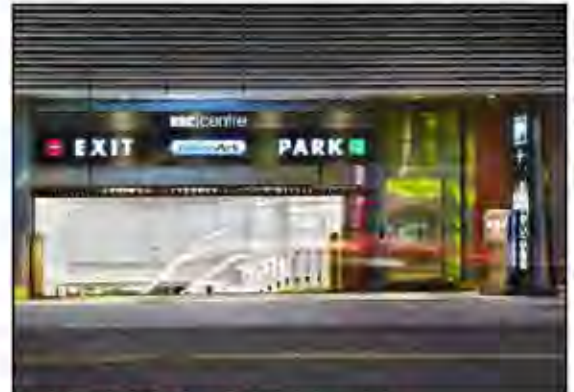
Figure 7.6: RBC Centre Parking Entrance
