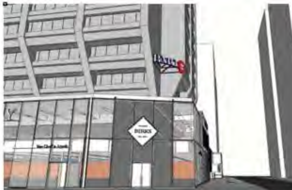
Figure 8.8: View of BCB-2 from Bloor Street at Bay Street
