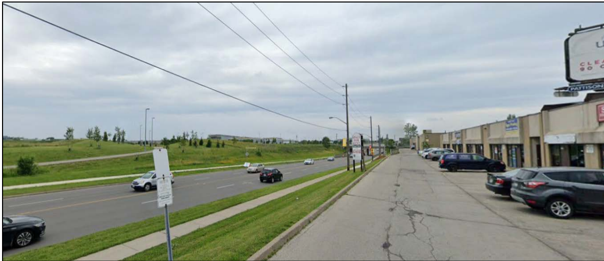
Figure 6 – Looking west from the Subject Premises, along Sheppard Avenue West
