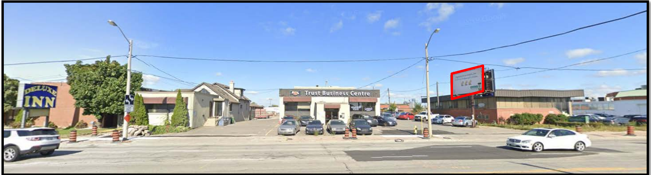
Figure 7: Google Street View of The Subject Premises- Looking North
