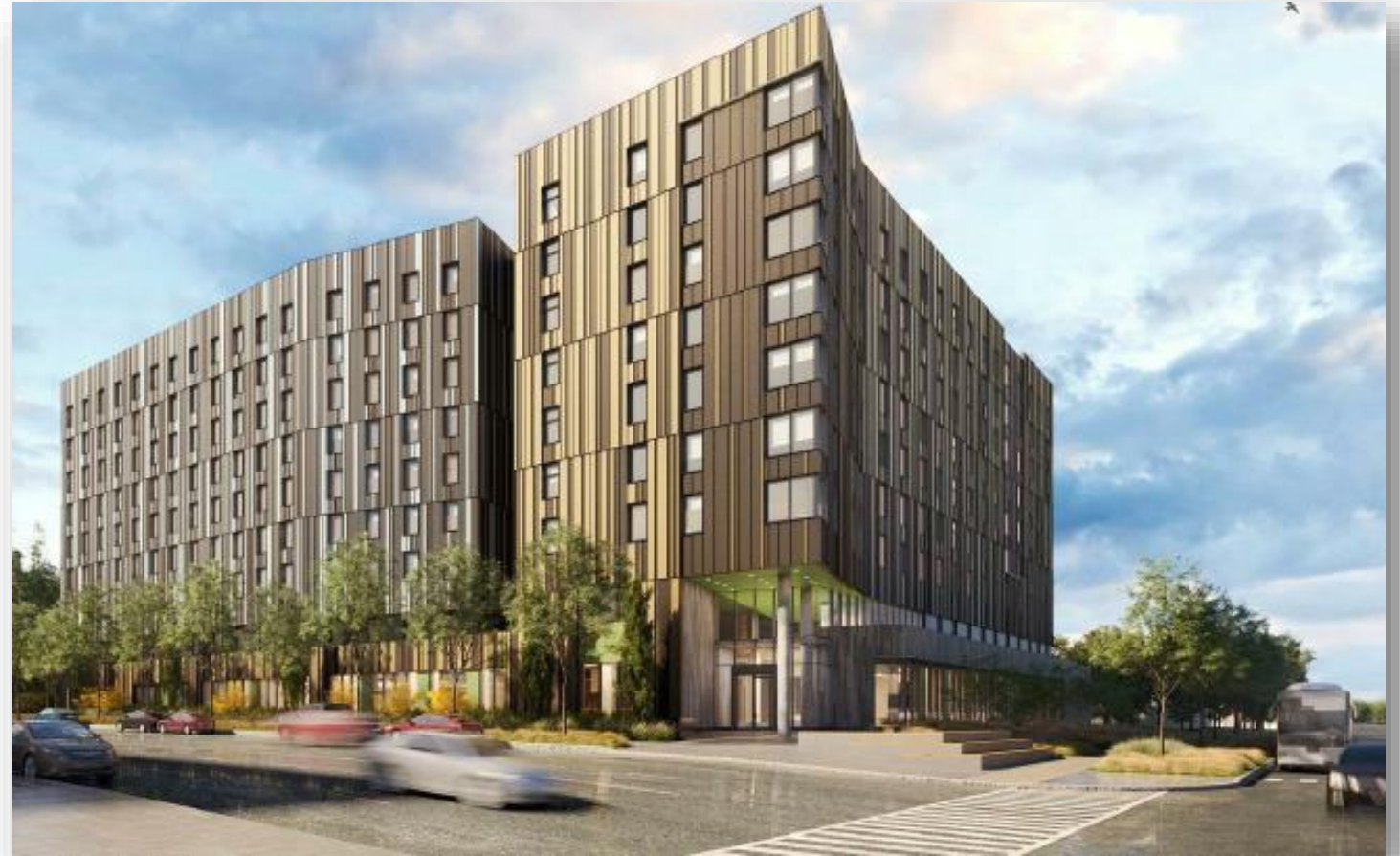
View from Ellesmere Road along realigned Military Trail (west façade) – Source: Core Architects, Handel Architects, LLP
