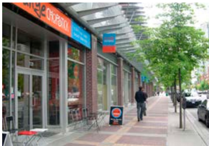
Columns/pilasters, canopy supports, sign bands, street trees, and paving patterns collectively contribute to a pedestrian friendly rhythm along a commercial street (Vancouver)
