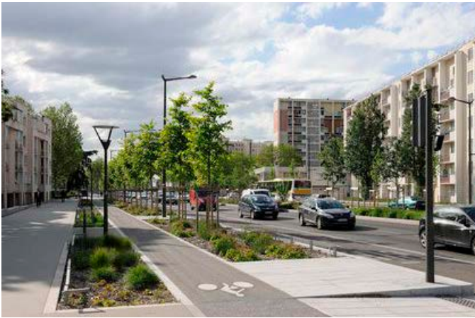
A generous boulevard with a cycle track with soft landscaping and trees on both sides (Lyon, France)
