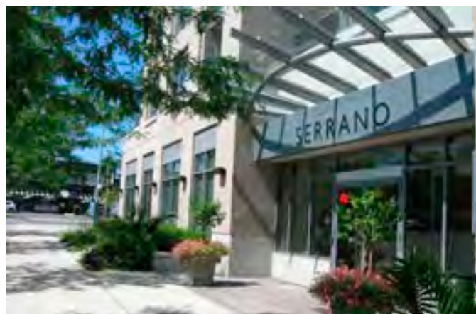
Tall and mid-rise buildings will have prominent main entrances fronting onto streets with features such as canopies and entry plazas with enhanced landscaping (Dunbloor Road, Toronto)
