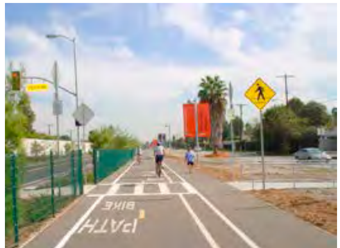
Multi-Use Path in Los Angeles, California, USA
