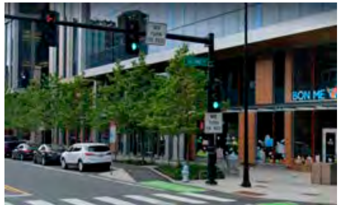
A cycle track integrated with street trees in the sidewalk zone (curb to building face) and on-street parking, adjacent to a mixed use development with commercial use at grade (Cambridge, Massachusetts, USA)
