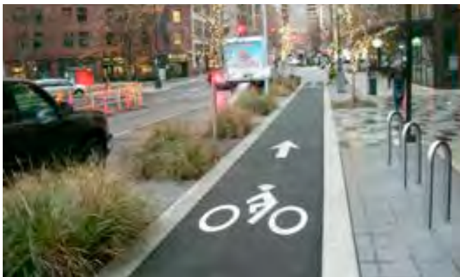
A safe cycling environment with a cycle track located at the same level as the sidewalk and separated from vehicular traffic (Seattle, Oregon, USA; Photo: theurbanist.org)
