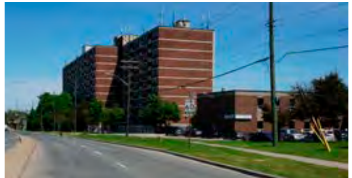
Birchmount Road and Eglinton Avenue East, looking north
