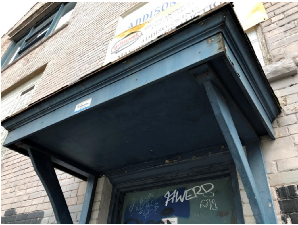
25. 41 Wabash Avenue: door canopy, main entrance, north elevation (HPS, 2020)
