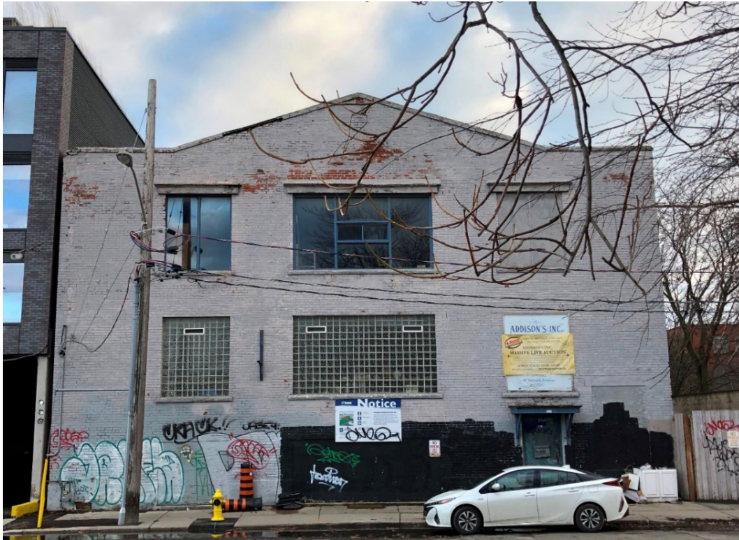
Photograph of the property at 41 Wabash Avenue (Heritage Preservation Services [HPS] 2020)
