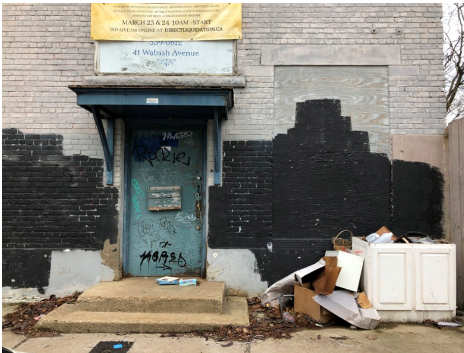
24. 41 Wabash Avenue: main entrance and Loading Bay, north elevation (HPS, 2020)
