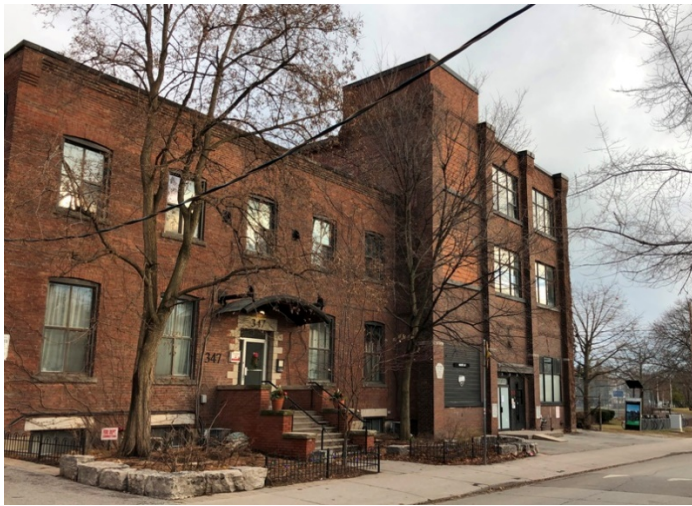
5. Former Chapman Double Ball Bearing Co., 1906, 345-347 Sorauren Avenue (HPS, 2020)
