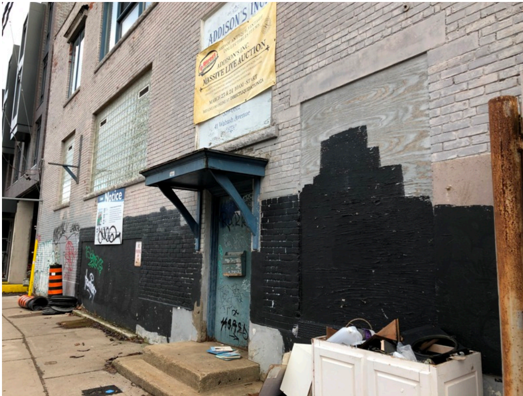
23. 41 Wabash Avenue: Detail of the north elevation entrances, and openings. (HPS, 2020)
