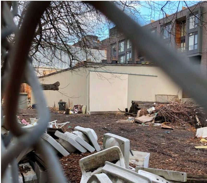
30. 41 Wabash Avenue: West and south elevations showing the rear shed with a roof sloping in the opposite direction from that shown on 1982-3 permit drawings indicating a possible recent replacement (HPS, 2020)
