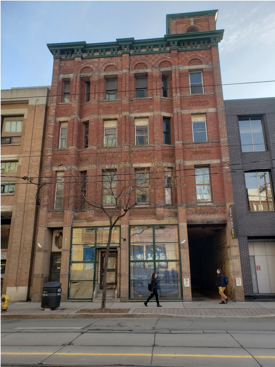
North Elevation of the Nealon House as viewed from the opposite side of King Street East
