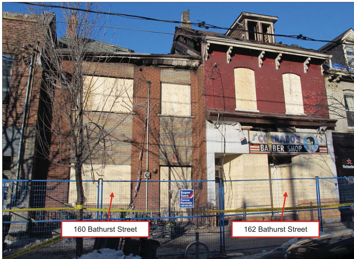
Figure 1: View of east elevation of subject building
