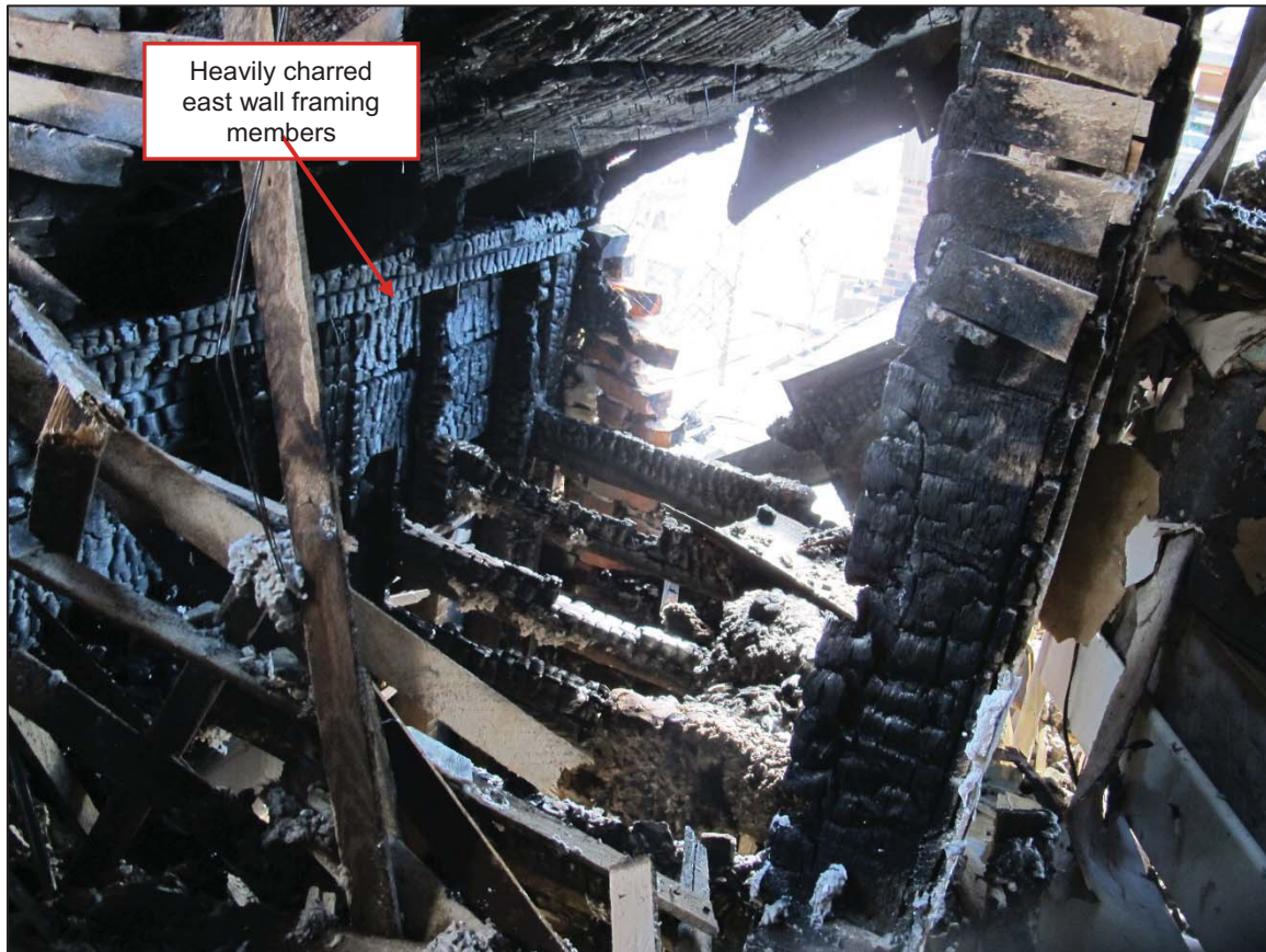
Figure 17: View of southeast corner of third level showing fire damaged framing members
