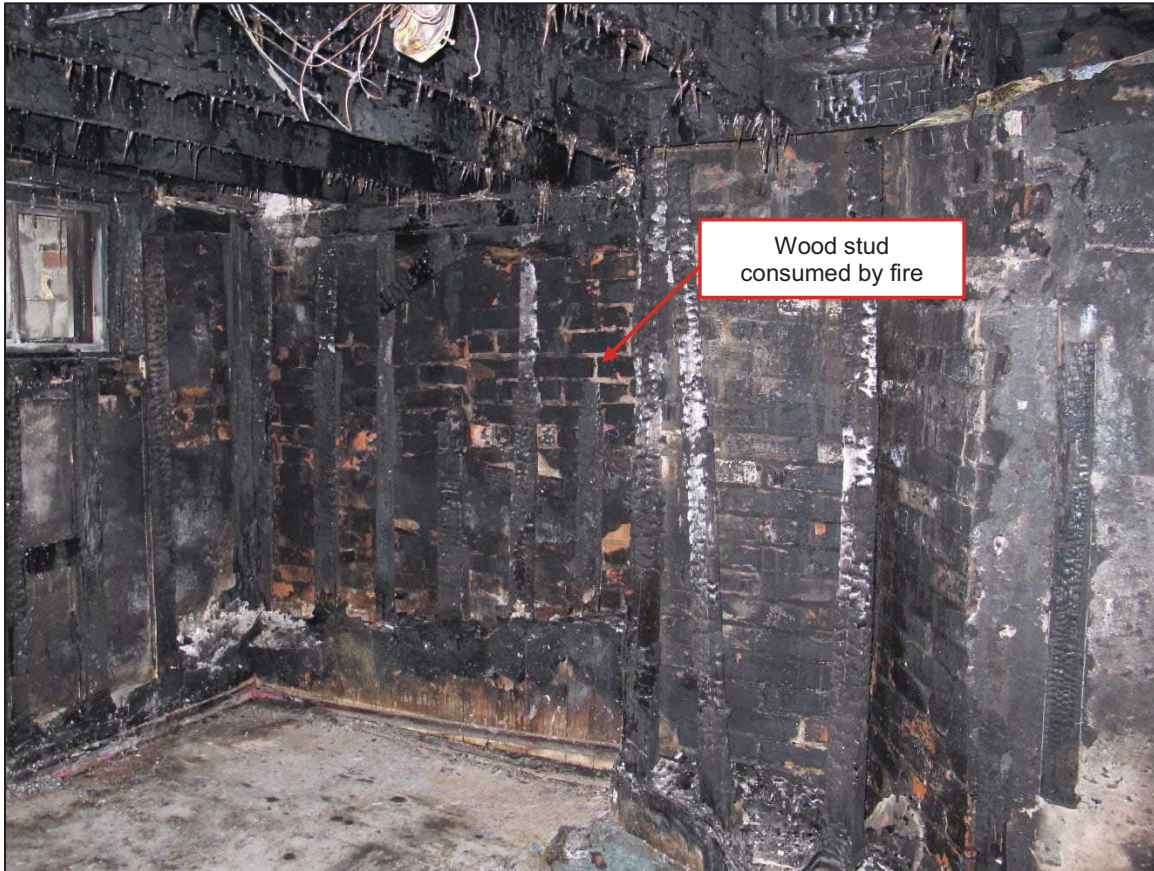
Figure 7: View of east end of south wall in basement showing charred wood studs and wall framing
