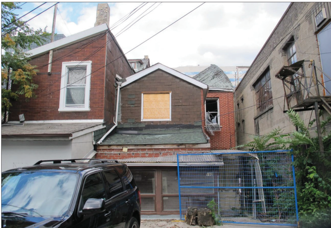
Figure 2: View of rear elevation of building showing secured condition
