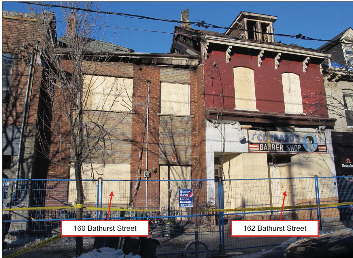
Figure 1: View of east elevation of subject building
