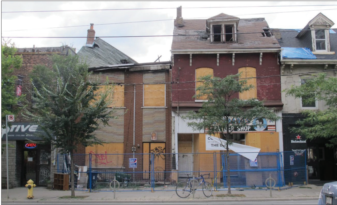
Figure 1: View of front elevation of buildings showing secured condition
