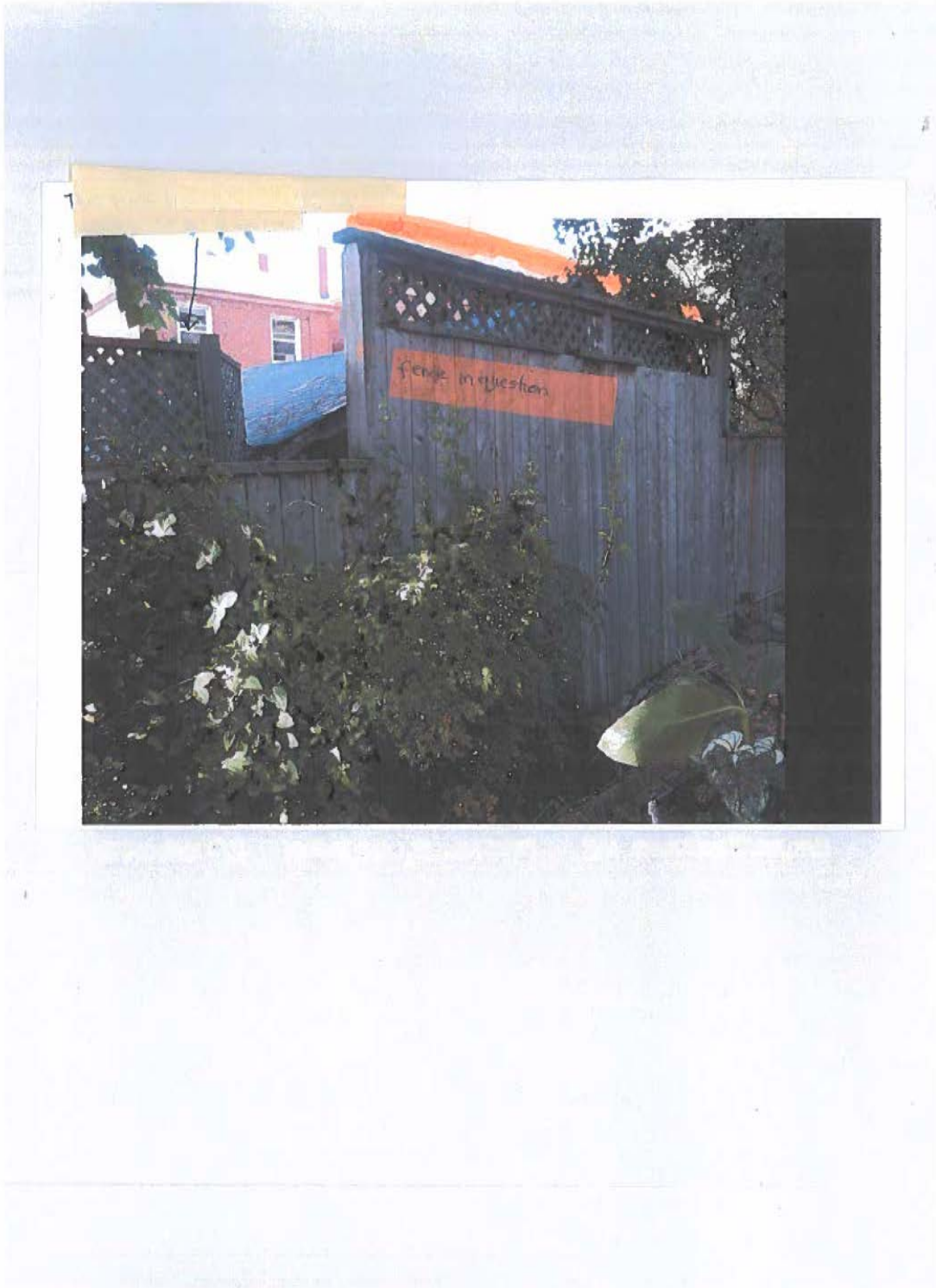
Appendix 2 North side rear fence 361 Monarch Park Avenue
